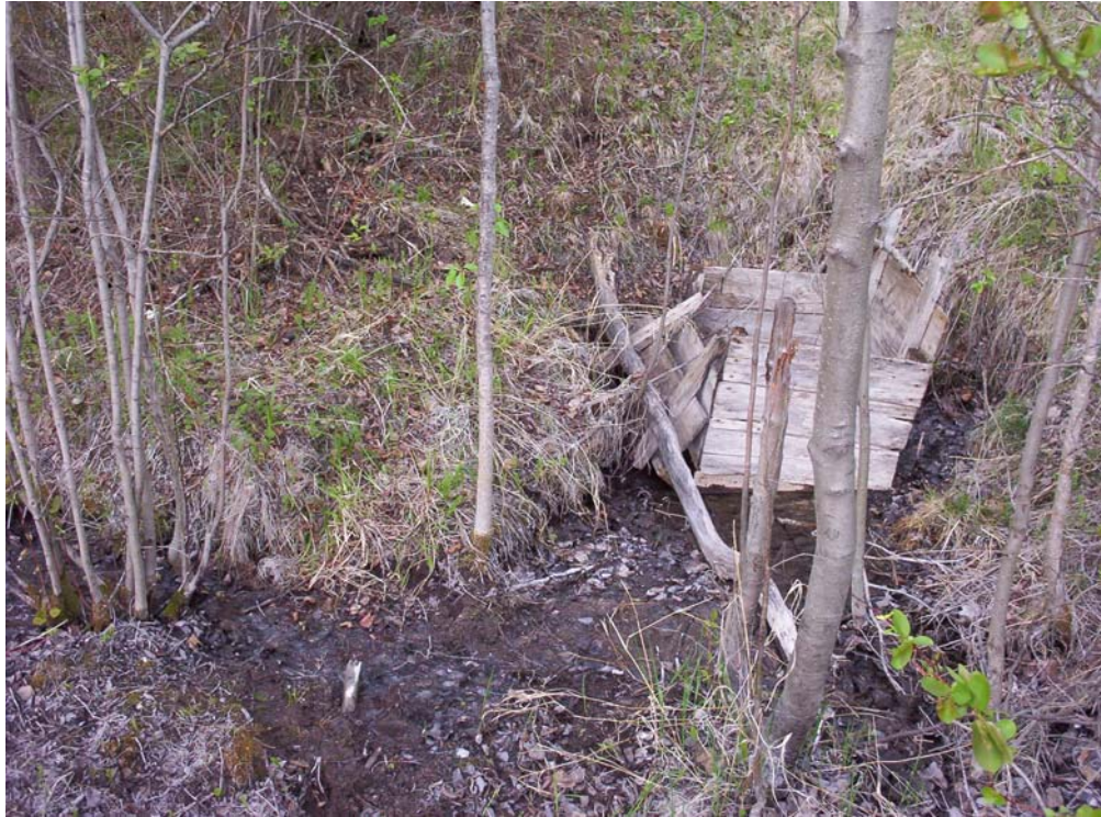
Spring at old wood casing well.
