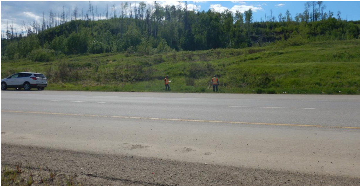
Photo No. 2 – Looking west at NC017A-2 landslide area
