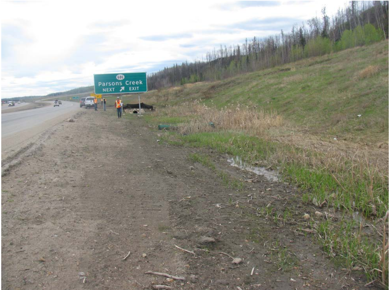
Photo 11 – Water ponding in the ditch (Looking South)
