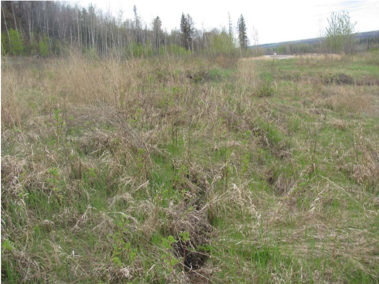
Photo 9a – Looking north at a relatively fresh head scarp crack of the lower backslope landslide
