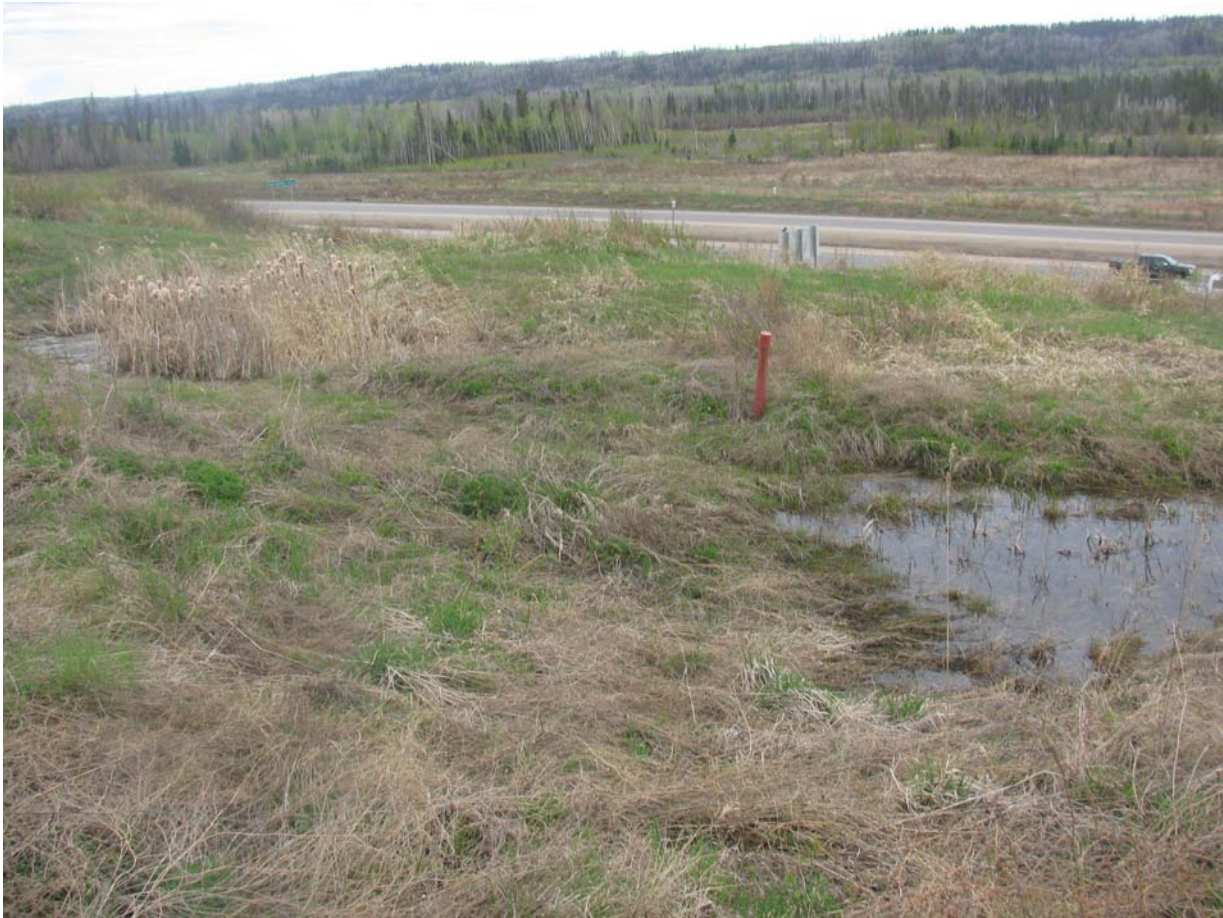
Photo 9 – Sag Ponds around PB09-2 within the lower backslope landslide mass (looking north); note that cattail vegetation has grown in one of the sag ponds
