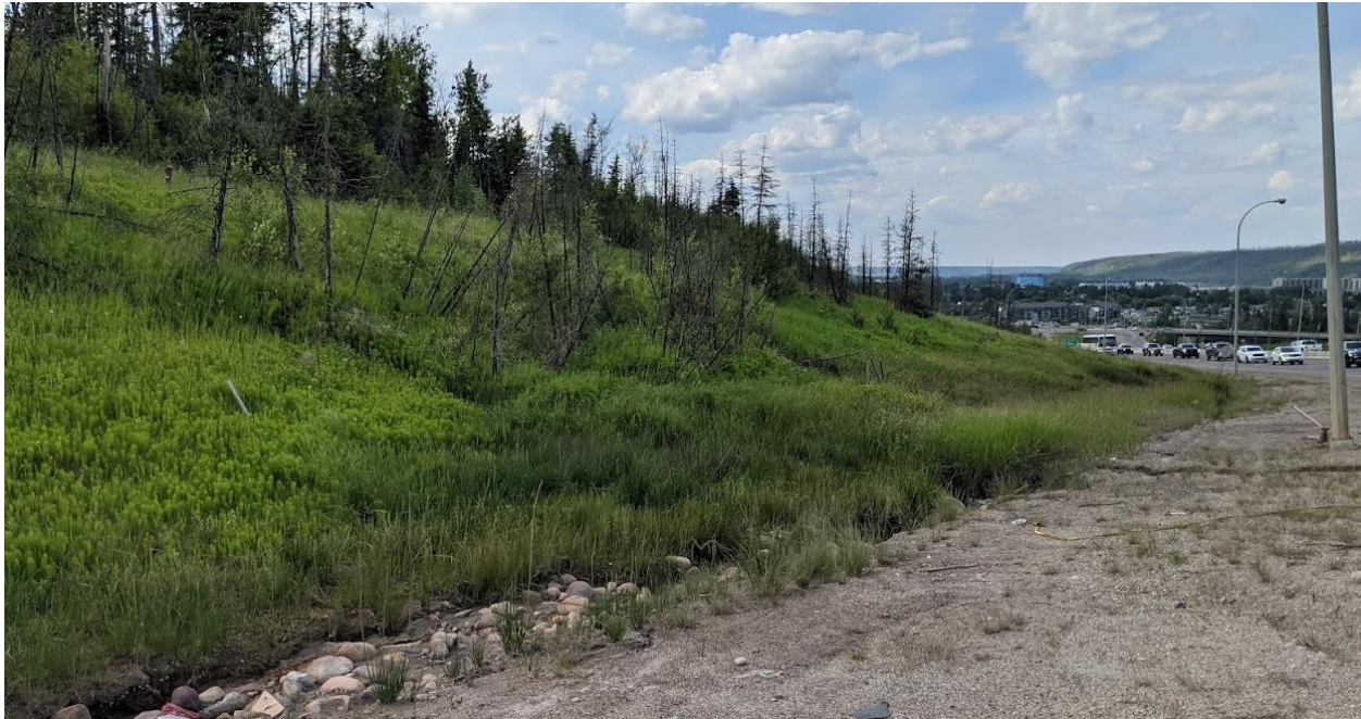
Photo No.1 – Looking north at the toe of the landslide; the landslide is toeing out above the ditch near culvert C6
