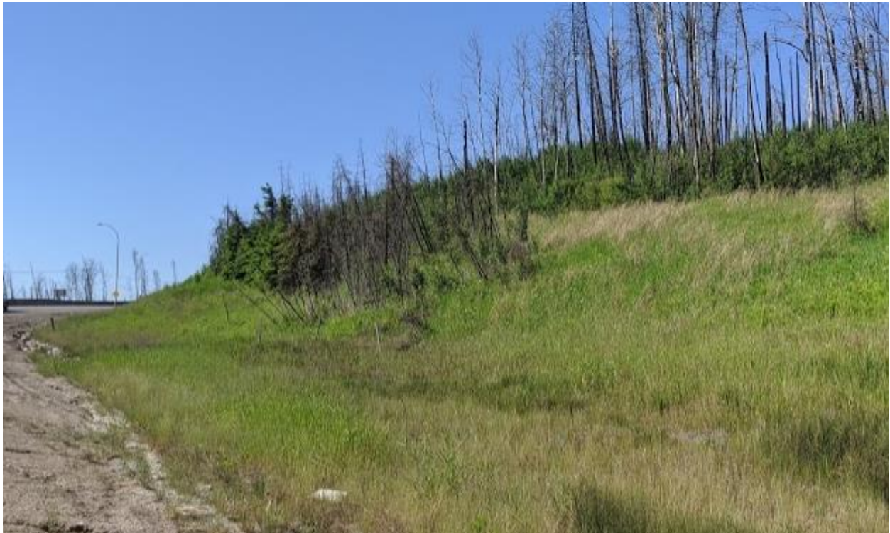
Photo No.3 –Looking south at the toe of the landslide; note tilting trees within the landslide mass
