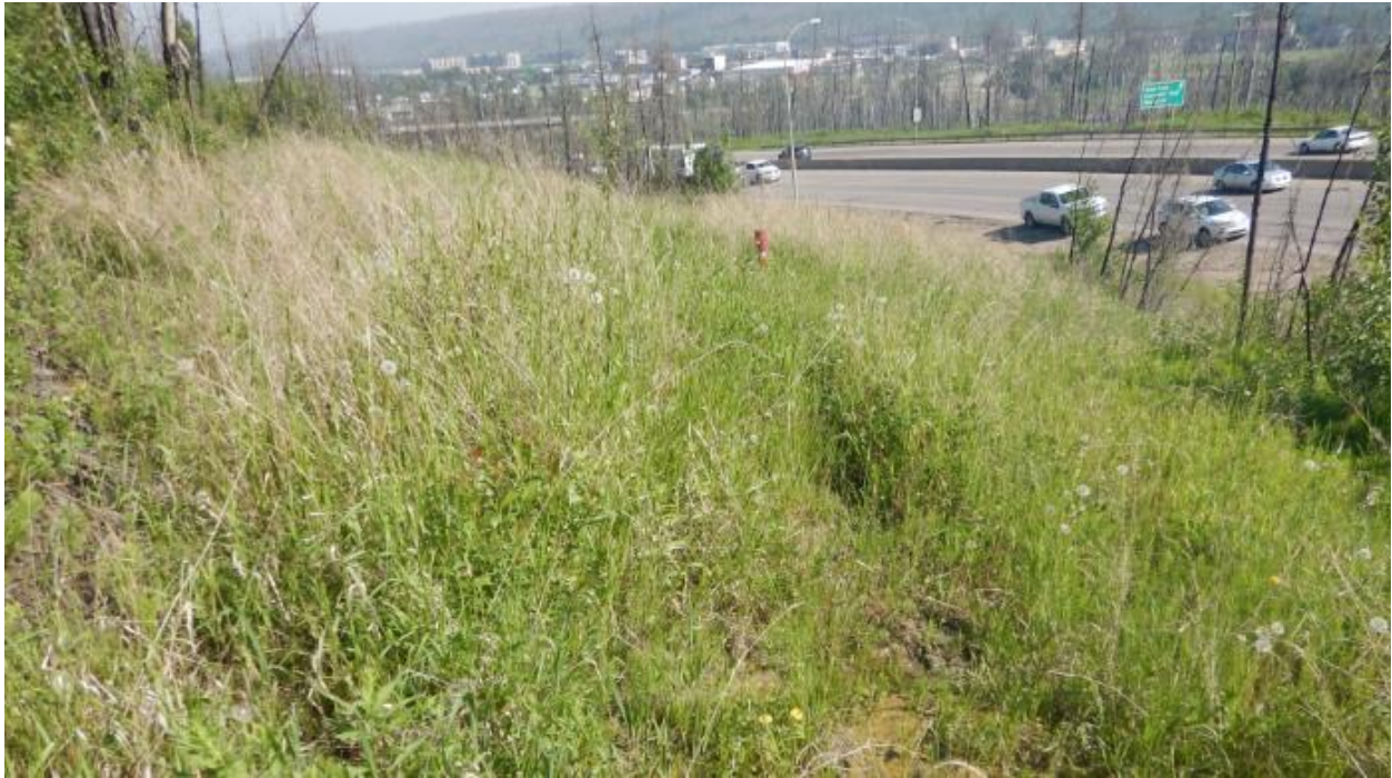
Photo No.4 –Looking north at S117-4; landslide mass is well vegetated
