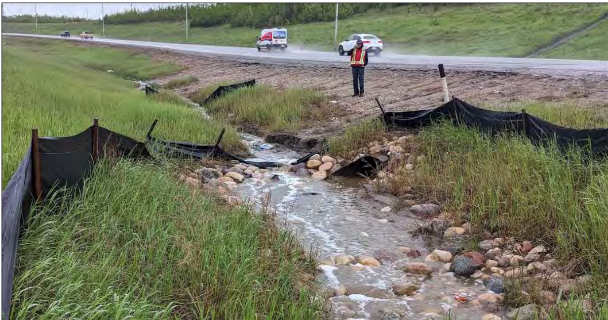
Photo 2 – Looking at the outlet of the 900 mm diameter SWSP culvert (C5a replacement);
