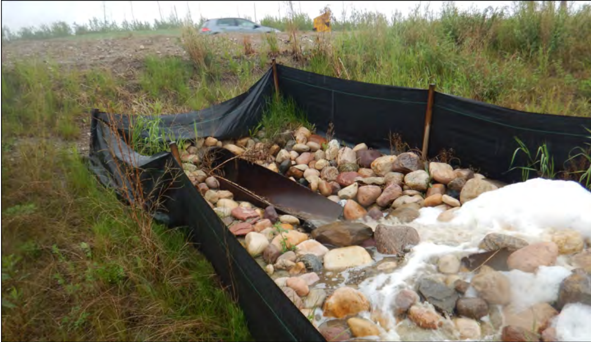
Photo 5 – Looking at the outlet of the C5b liner.
