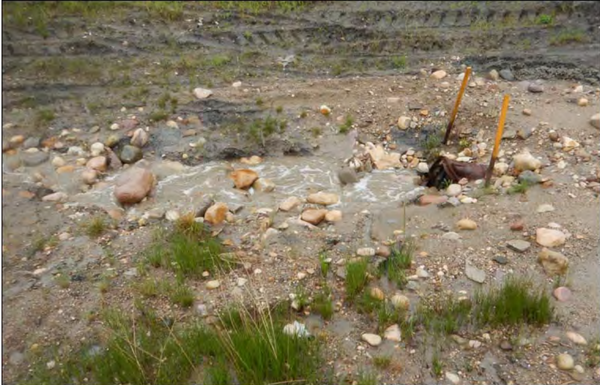
Photo 9 – Culvert C6 inlet previously buried under sediment was exposed in 2024
