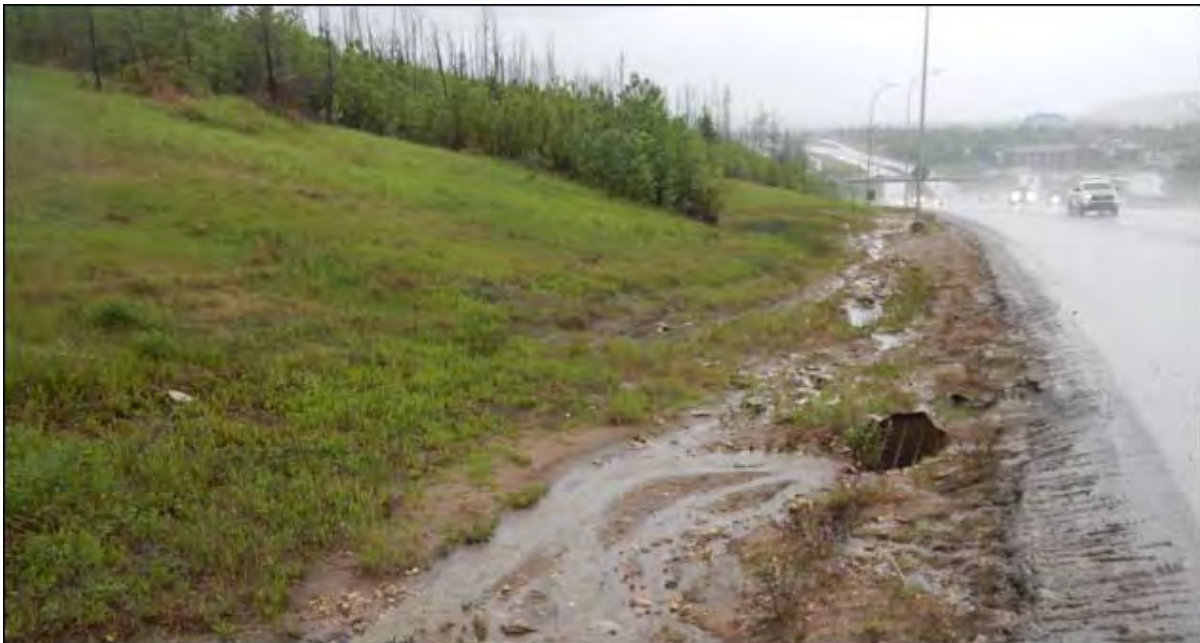
Photo 10 – Drop structure DS2 exposed in 2024
