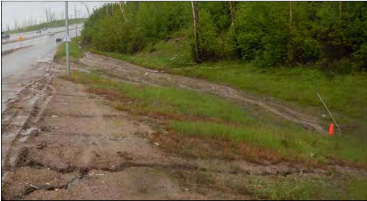
Photo 15 – Drop Structure DS1 exposed in 2024
