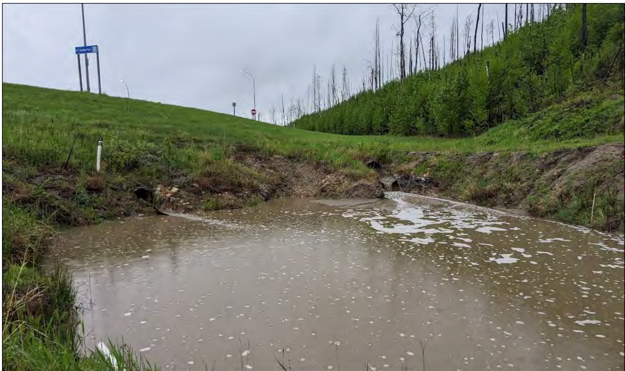
Photo 18 – Culvert C3 and C4 outlets
