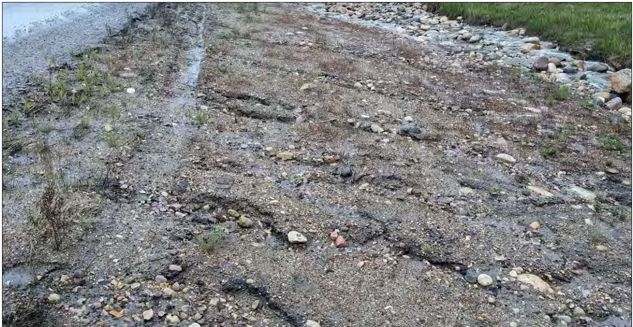
Photo 8 – Bare side slopes with minor erosion rills (looking south)
