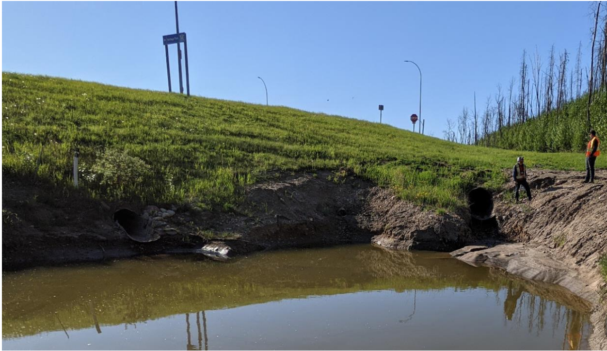
Photo 11 – Culvert C3 and C4 outlets; no flow from C3.
