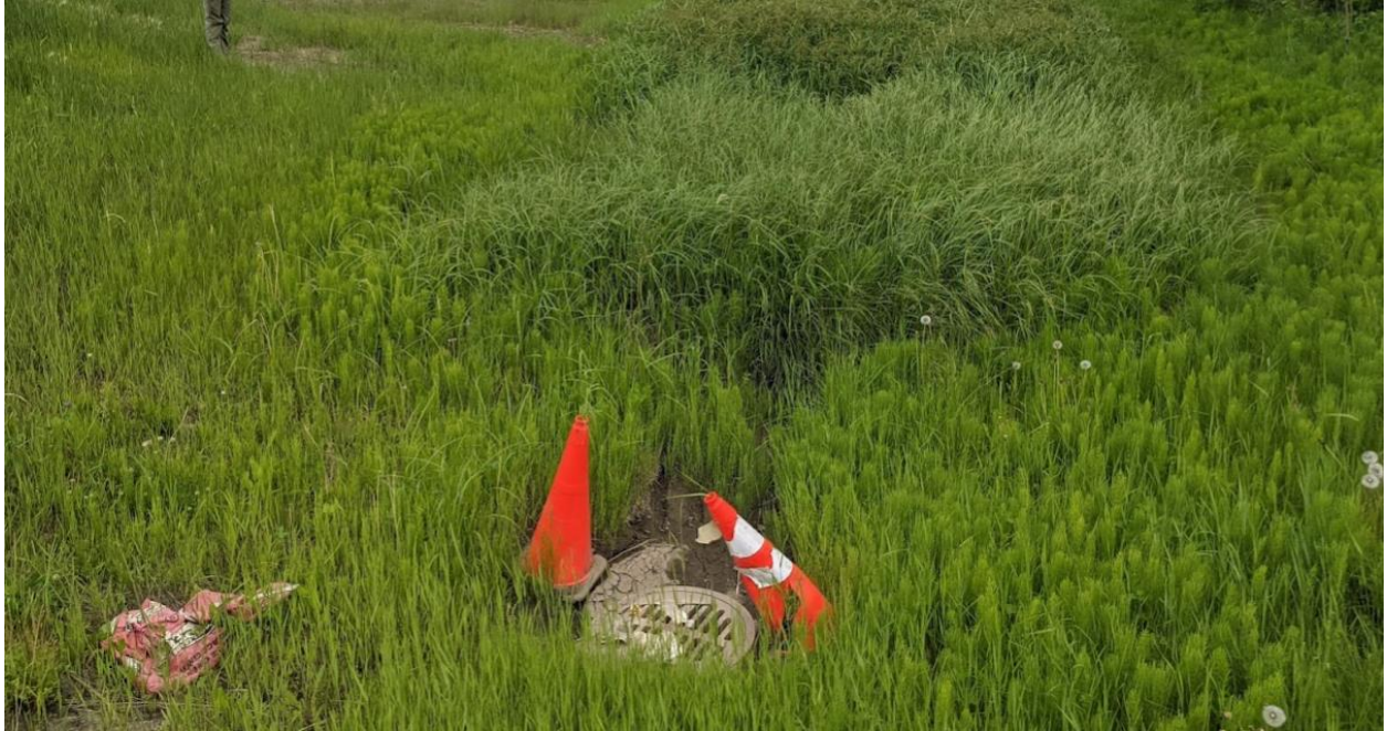
Photo 8 – Drop Structure DS1; note lush vegetation possible due to seepage and surface water flowing from the hill
