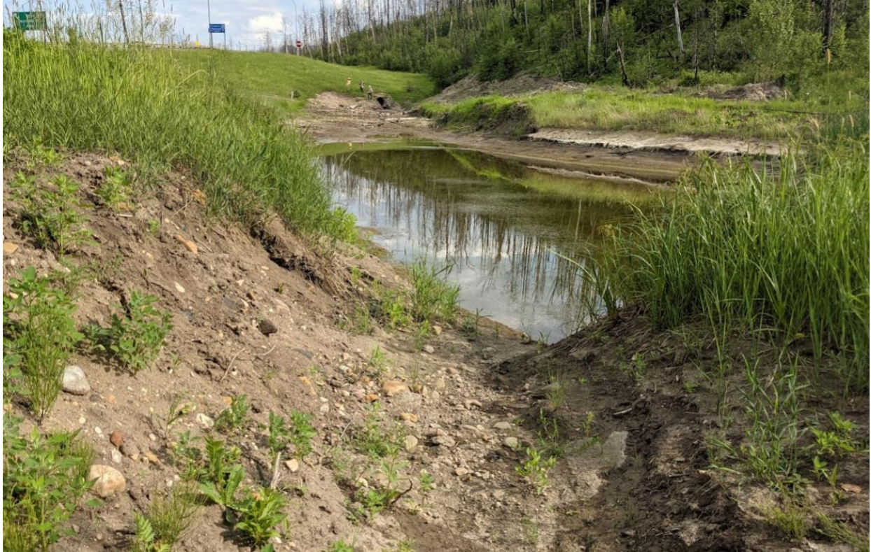
Photo 12 – Pond outflow discharge channel; approximately 0.5 m freeboard
