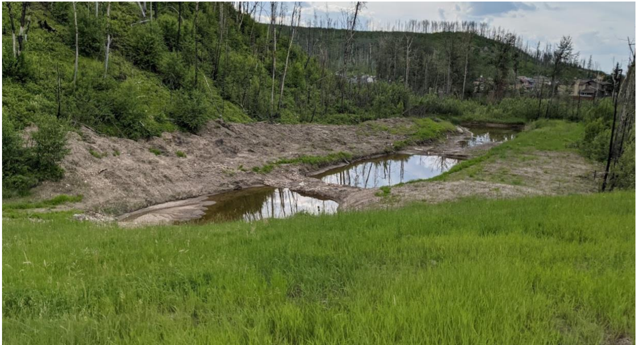
Photo 9 – Substantial sediment was removed increasing pond capacity by approximately 1.5m
