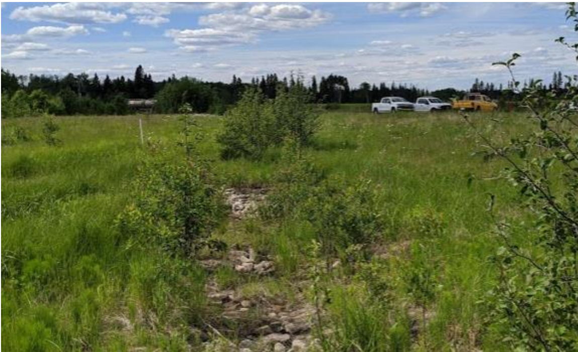
Photo No.2 – Looking west at the riprap-lined swale to the south of the TSA pad; minor water ponding within the swale
