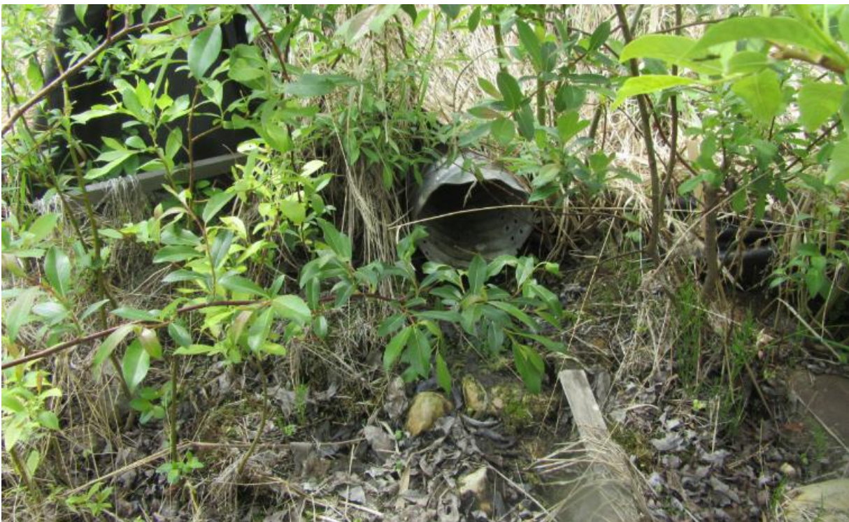
Photo No.10a – Subdrain S4; no flow observed
