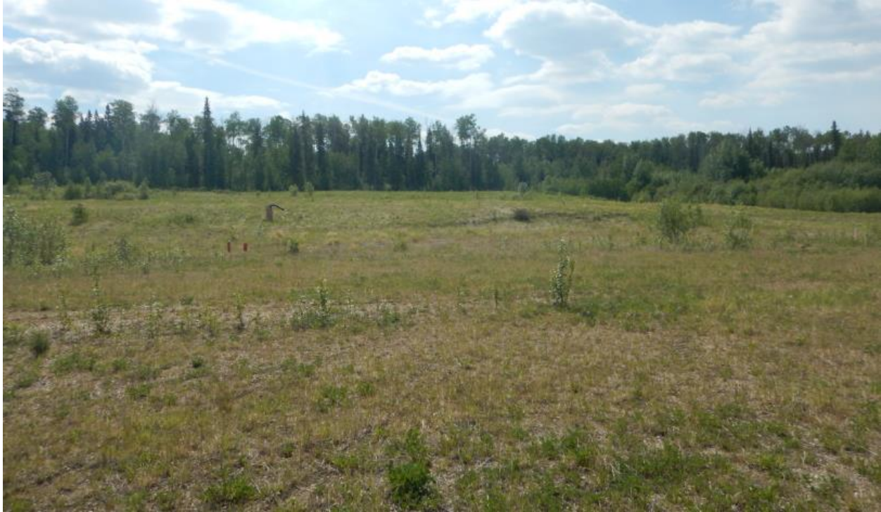
Photo No.1 – West landslide vegetated head scarp crack (Looking South)
