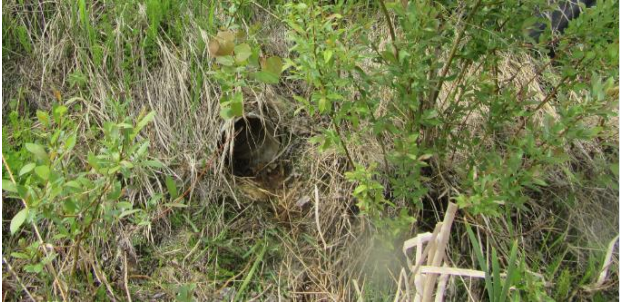
Photo No.11 – Subdrain S3; no flow observed
