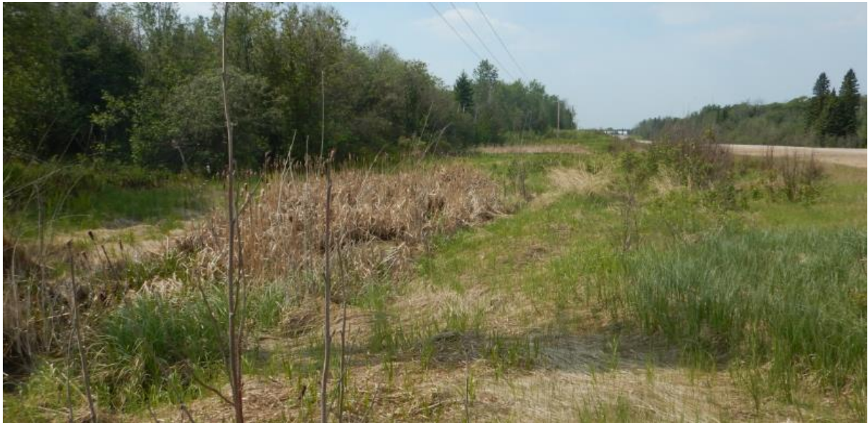
Photo No.4 – Looking at highway south ditch to the west of the TSA pad; note standing water and cattail vegetation (Looking West)
