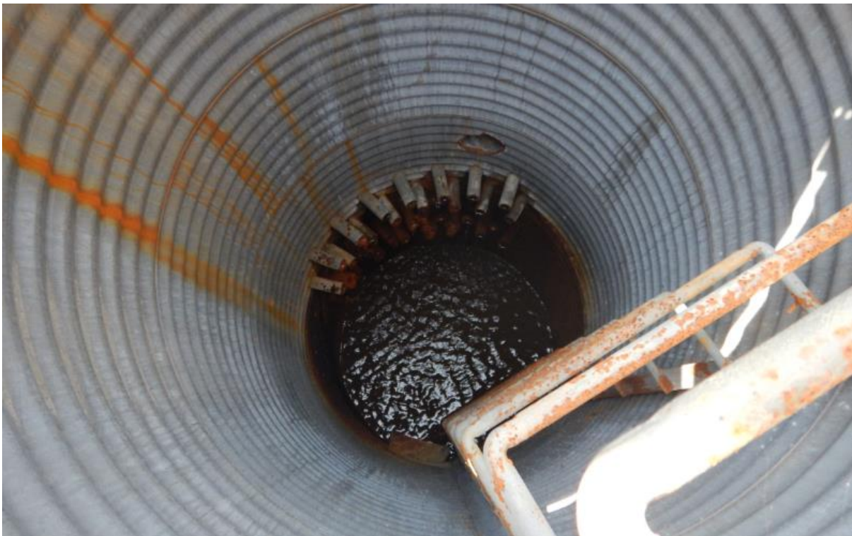
Photo No.6 – Manhole 1; note water flowing from sub-horizontal drains
