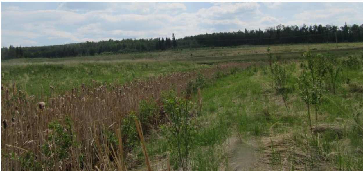
Photo No.12 – Water Ponding within the riprap lined channel located between the east and west landslide berms (Looking South)
