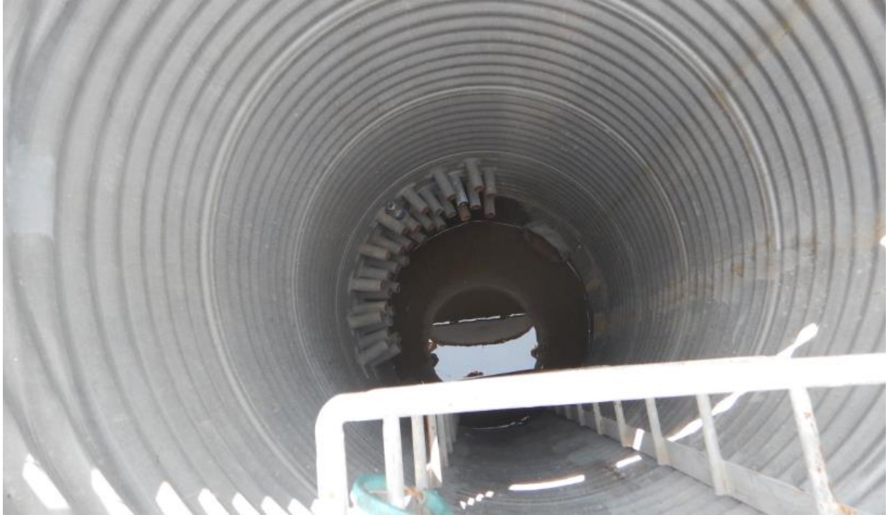
Photo No.7 – Manhole 2; no water was observed
