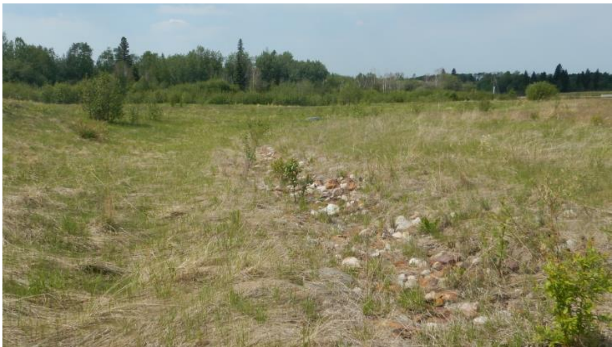
Photo No.2 – Looking west at the riprap-lined swale to the south of the TSA pad; minor water ponding within the swale
