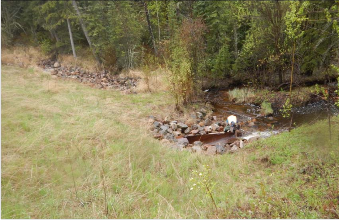
Photo No. 9 – SWSP outlet; note heavy water flow in 2024
