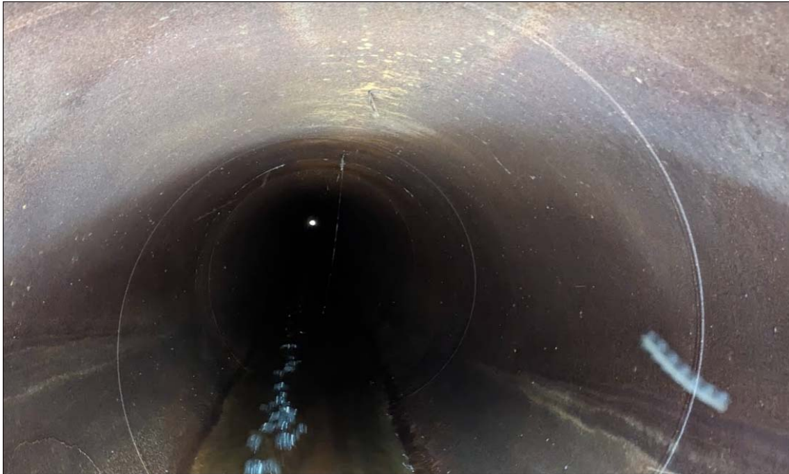
Photo No. 4 – SWSP Culvert Inlet inner condition
