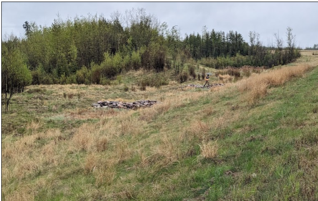
Photo No. 6 – Rock check dams located along NBL southeast ditch
