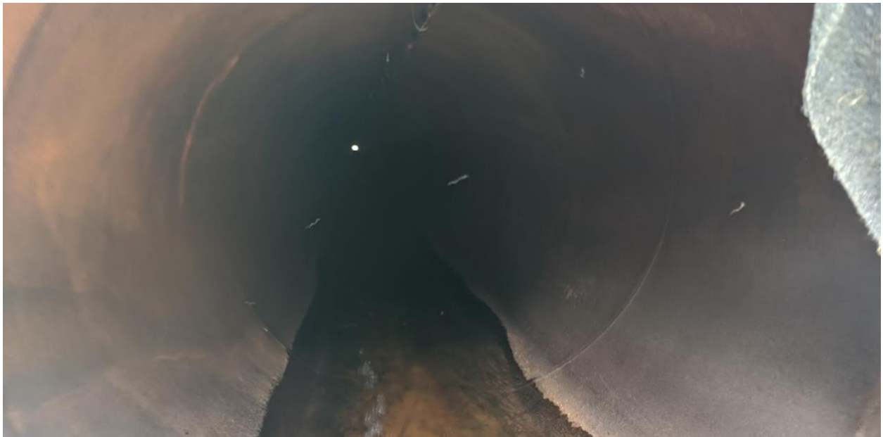
Photo No. 8 – Looking inside the SWSP culvert from inlet location
