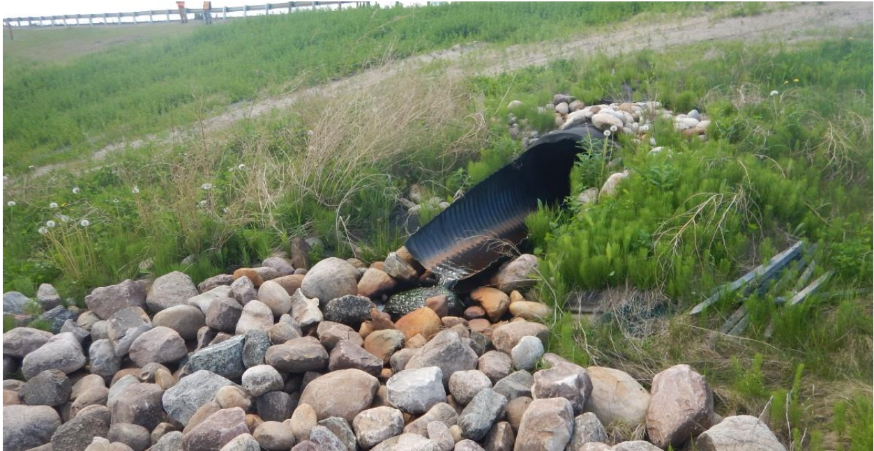
Photo No. 5 – CSP culvert C3 outlet
