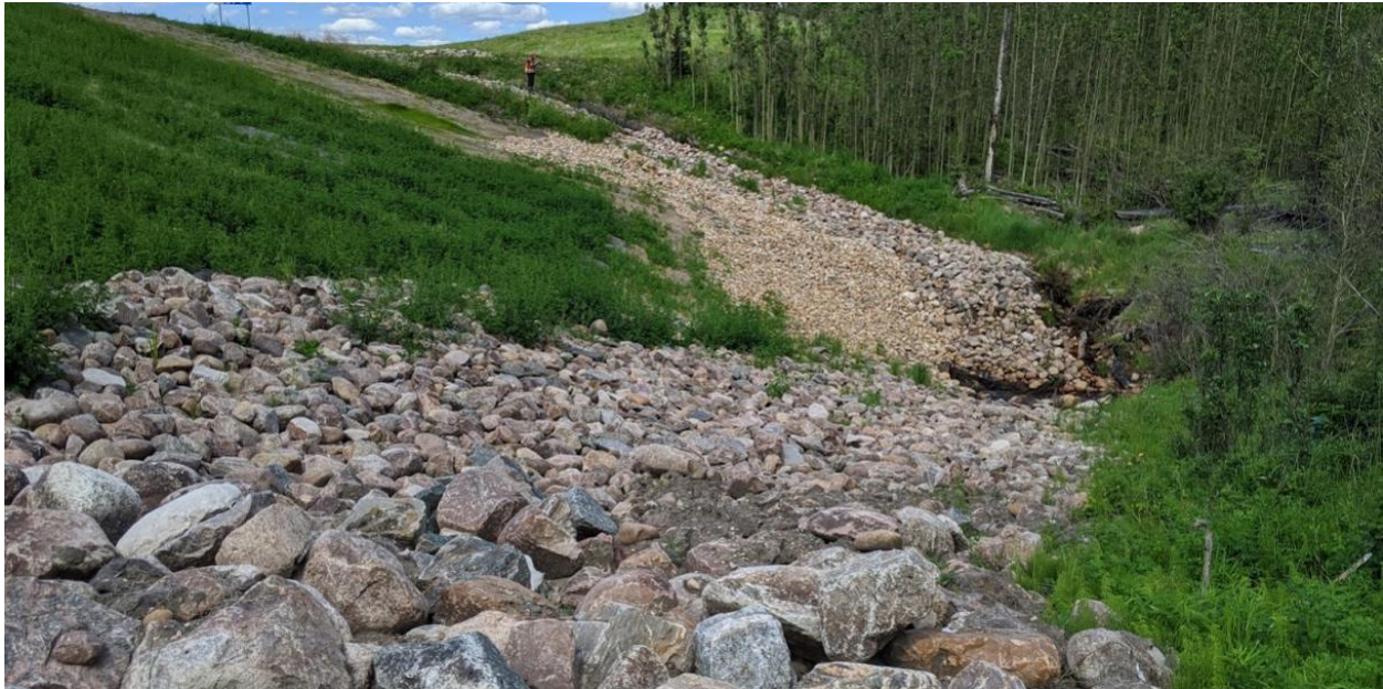
Photo No. 9 – NBL embankment east side slope; note poor vegetation growth upslope of the centre portion of the riprap
