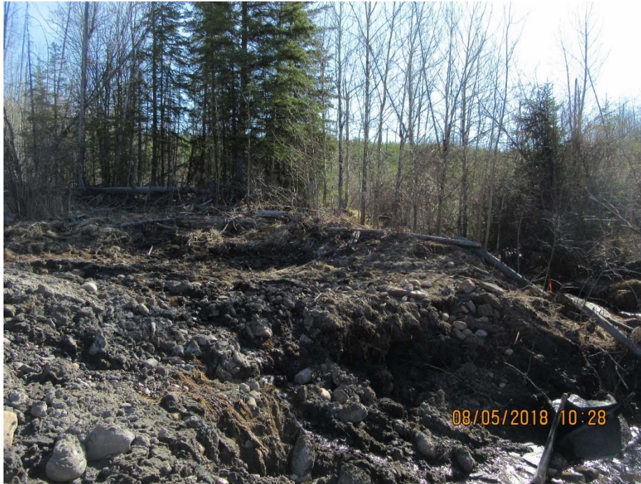
Photo No. 3 - Uncontrolled discharge of surface flow from the north channel into the slope (looking east)
