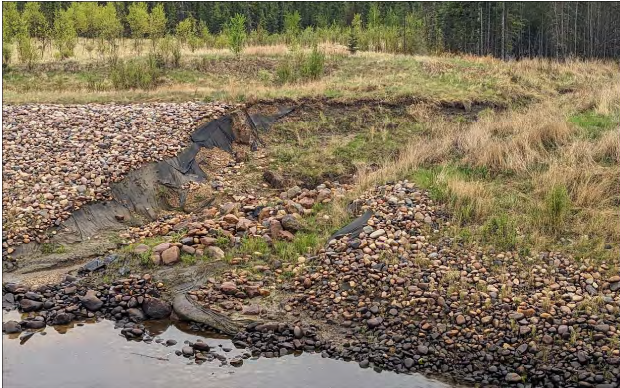
Photo No. 3 – Looking southeast at the same area in Photo No. 2
