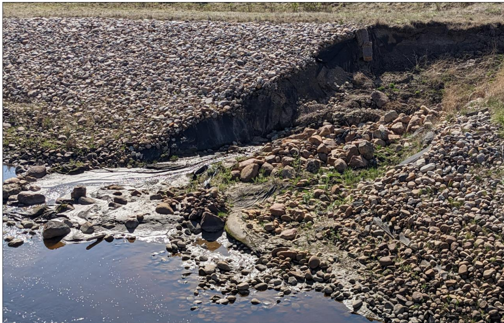
Photo No. 4 – Looking southeast at the same area in Photo No. 3
