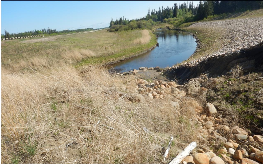
Photo No. 3 – Looking north at north facing riprap channel to the east of the bridge location. Note the deep erosion along the channel.
