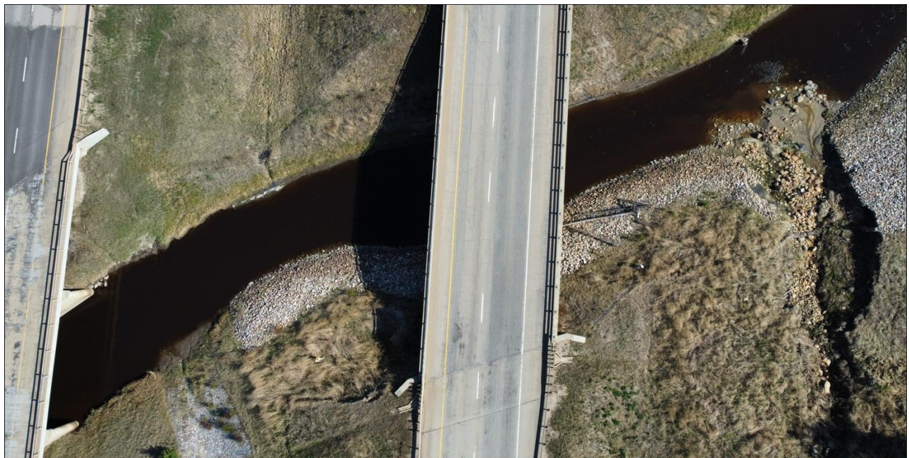
Photo No. A2 – Aerial view showing existing active slumps to the east and the west of the bridge south headslope and a severe erosion gully along the highway east ditch; both landslides reduced the stream width; note sediment accumulations within the stream at the mouth of the erosion gully.
