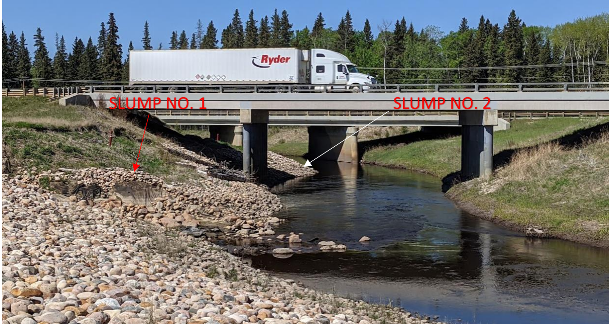
Photo No. 5 – Looking west at river channel; Note slumping within the riverbanks to the east (slump 1) and the west (slump 2) of the south headslope location and the distinct toe rolls in the river channel.
