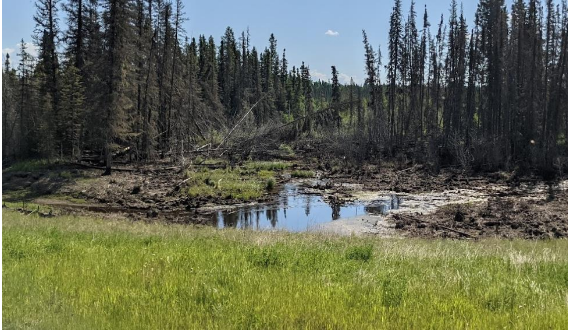
Photo No. 1 – Looking southeast from the south side of the bridge at the low lying area within the bush. This area was noted to be flooded in 2020, but it is currently drained due to beaver dam removal by AT in the fall of 2020
