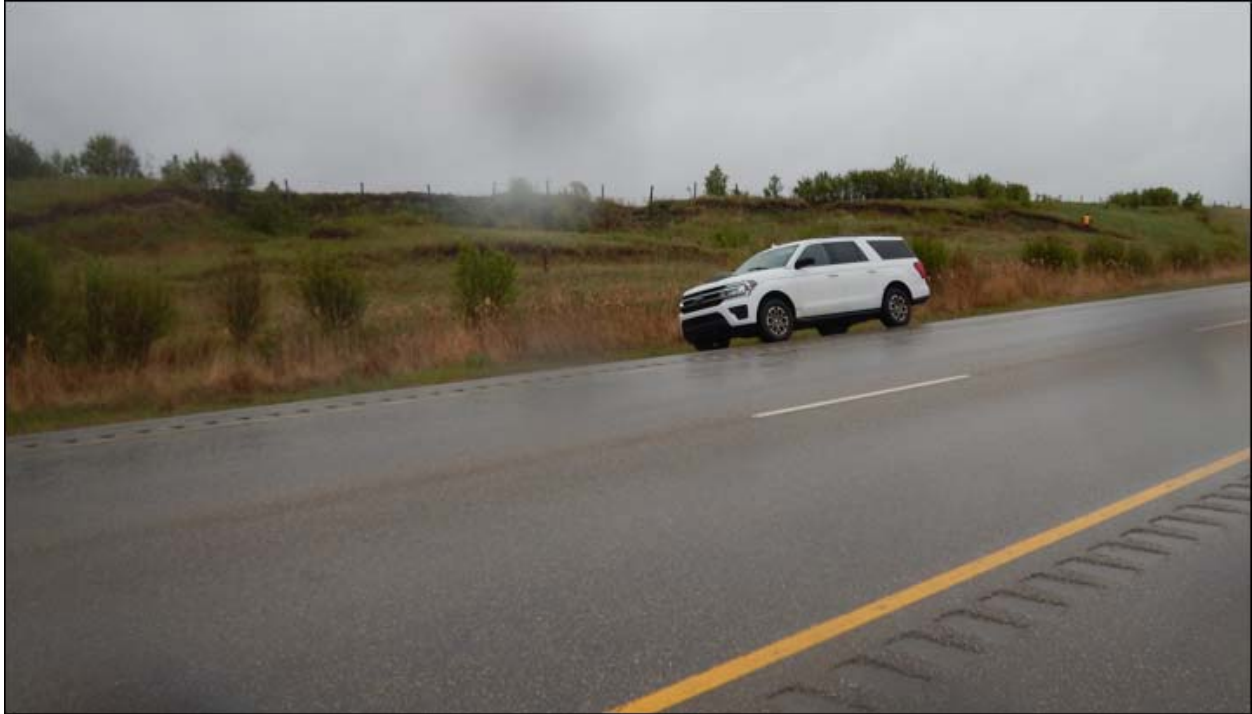
Photo No. 1- NC091-1: Looking southeast at the landslide area
