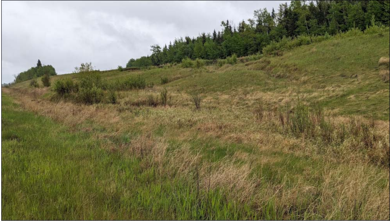
Photo No. 7 – NC091-2: Looking north at the landslide mass; note the presence of a distinct toe roll in the ditch
