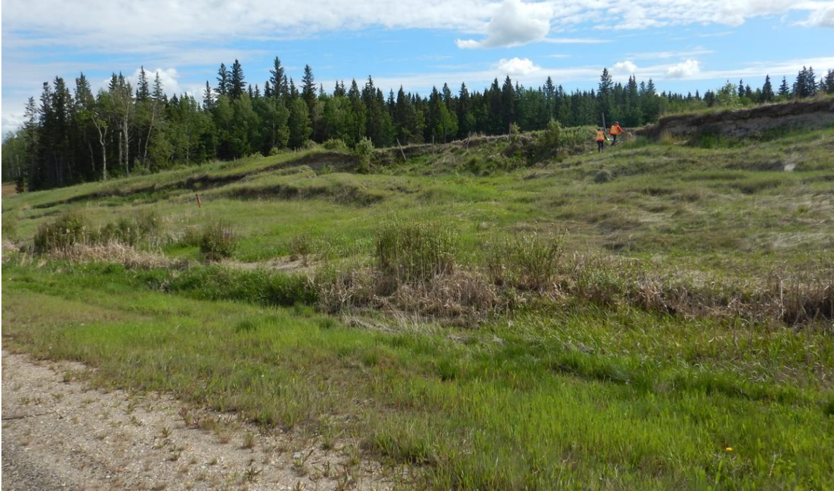
Photo No. 3- NC091-1: Looking northeast at the landslide mass; note the presence of multiple tension cracks in the slope and cattails in the highway ditch
