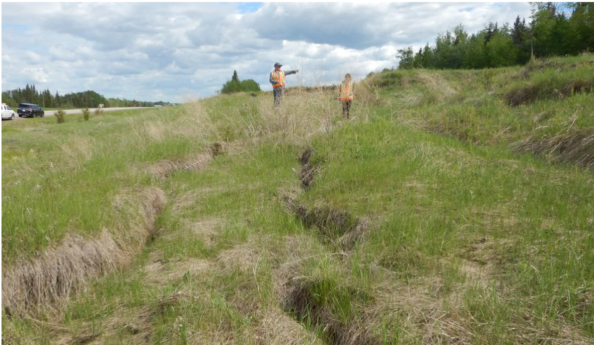
Photo No. 8– NC091-2: Looking northeast at the southern flank of the landslide mass; note the presence of multiple tension cracks within the backslope
