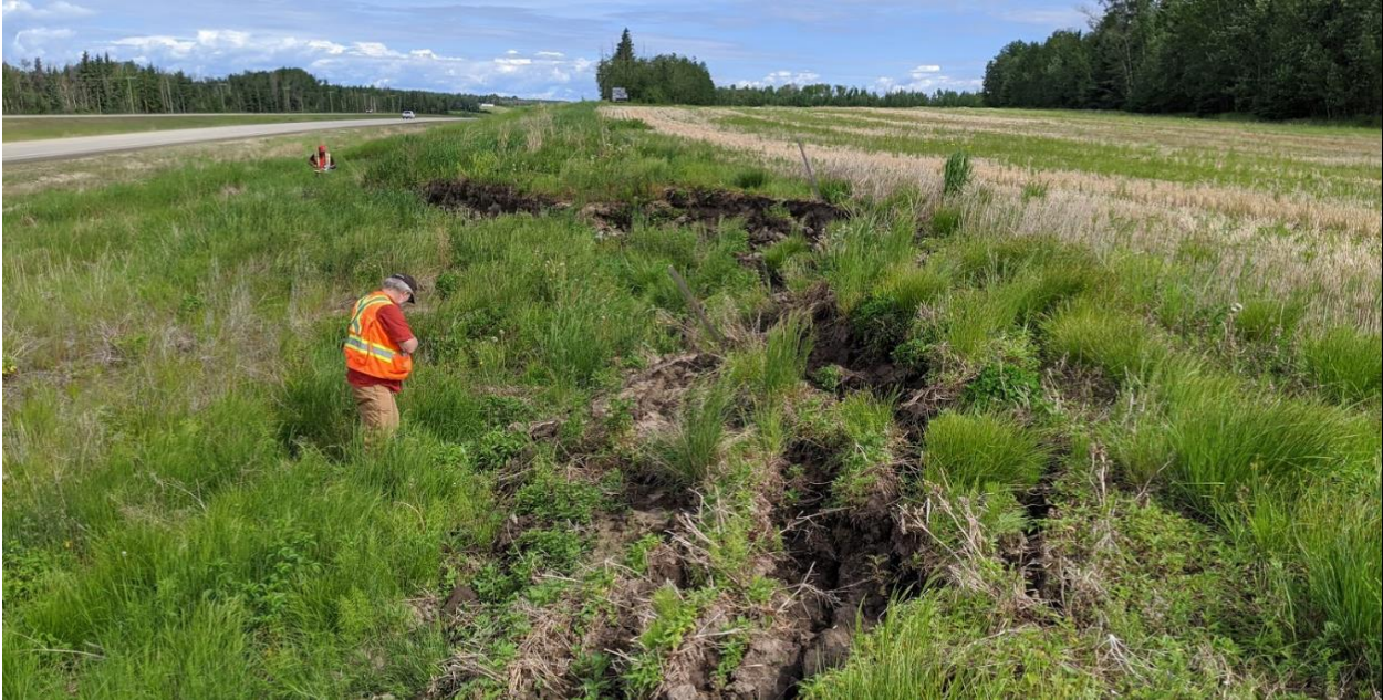
Photo No. 11 – NC091-2: The second portion of the scarp that cuts into the adjacent field (north portion).
