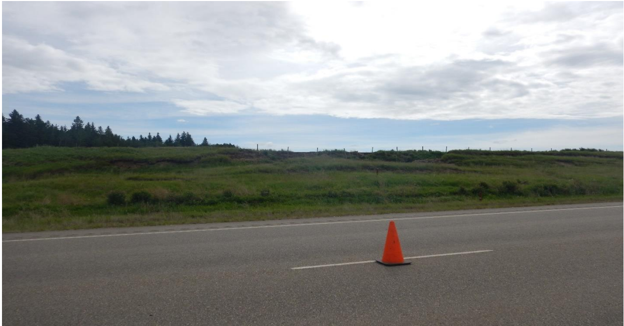
Photo No. 2a- NC091-1: Looking east at the landslide mass
