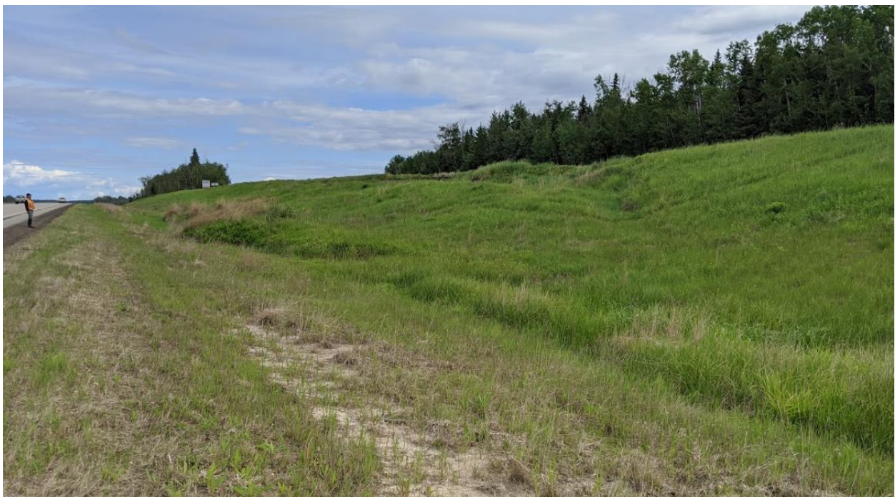
Photo No. 7 – NC091-2: Looking north at the landslide mass; note the presence of a distinct toe roll in the ditch
