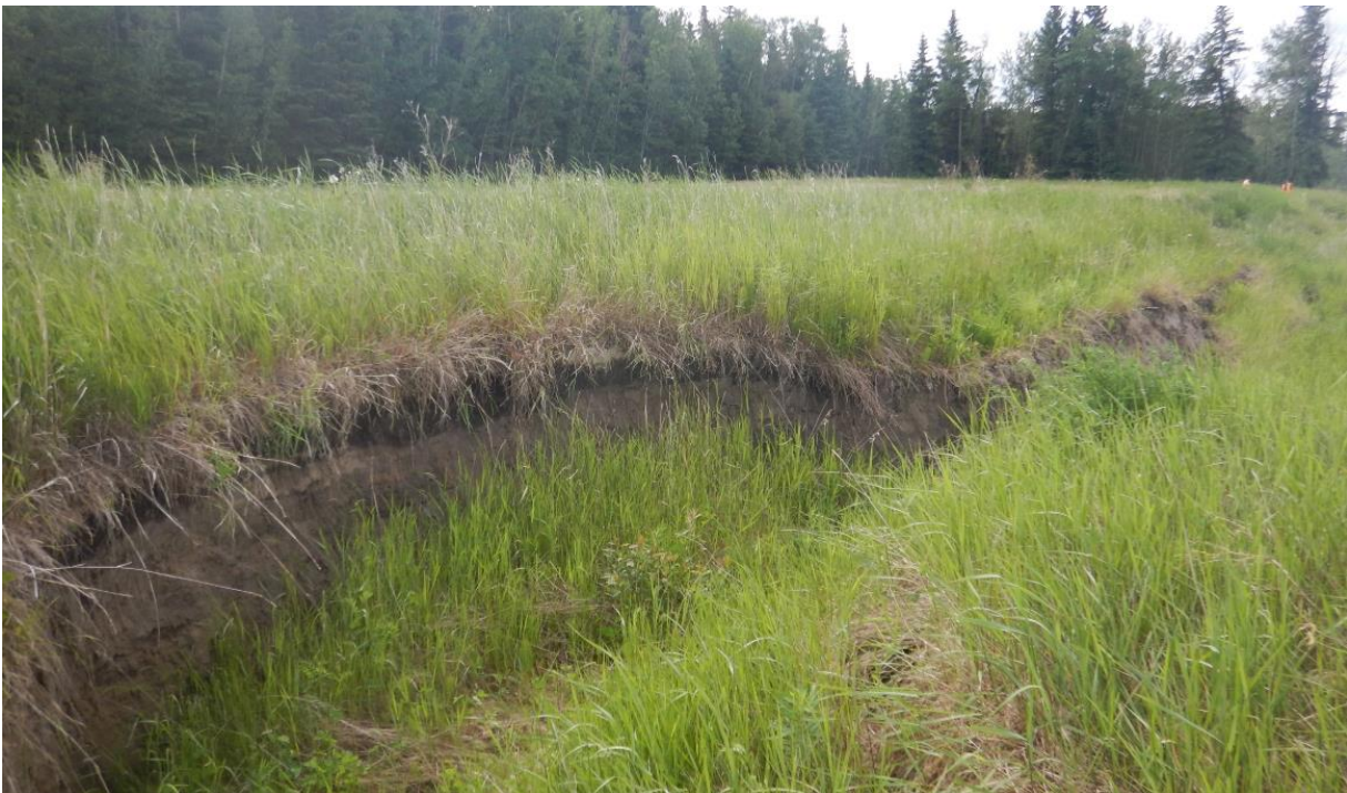
Photo No. 8 – NC091-2: Exposed sandy soils at main scarp.
