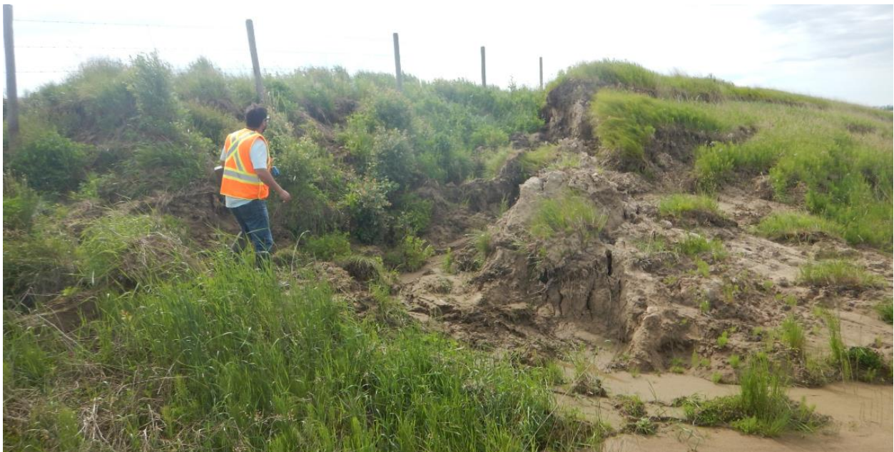
Photo No. 5 - NC091-1: Looking southeast at exposed sandy soils of backslope.
