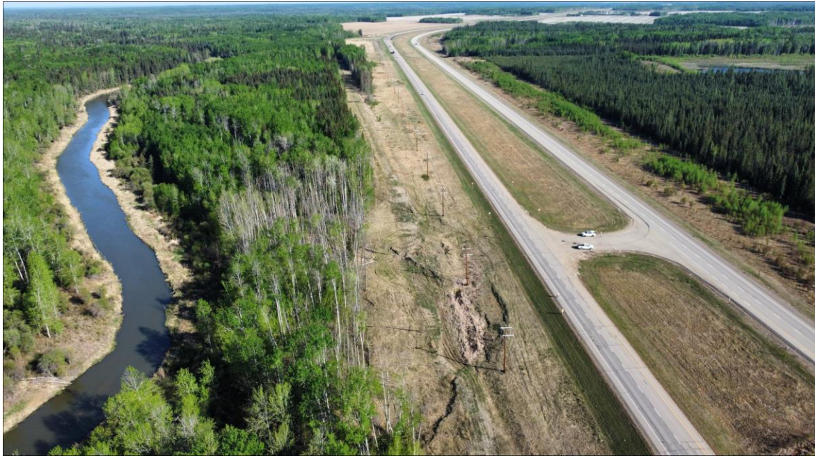
Photo No. A5 (aerial photo) – Looking north at the active landslide mass to the west of Hwy 63. Note head-scarp crack between the edge of pavement and power lines, fresh quad tracks within Fischer trail, dead/tilting trees within landslide mass, and toe of the landslide narrowing of the river channel at the river bend.
