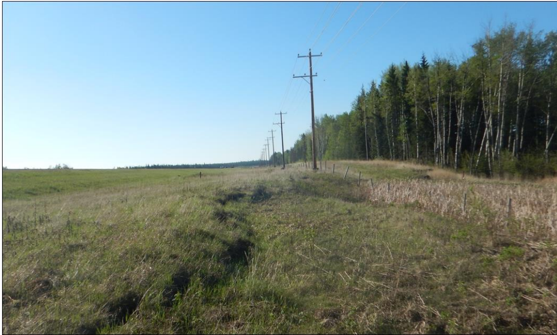
Photo No.3 – Looking south at the southern flank of the landslide (700 mm wide cracks, up to 1 m drop); water ponding along the ditch between the trail and the fence (note cattails in this area)
