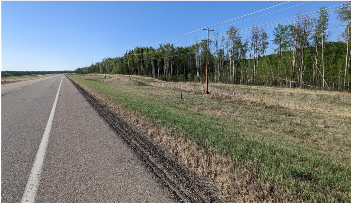
Photo No. 7 – Looking south at highway southbound lanes; landslide is not currently impacting the highway surface; head scarp crack is about 6.5 m away from the edge of pavement.
