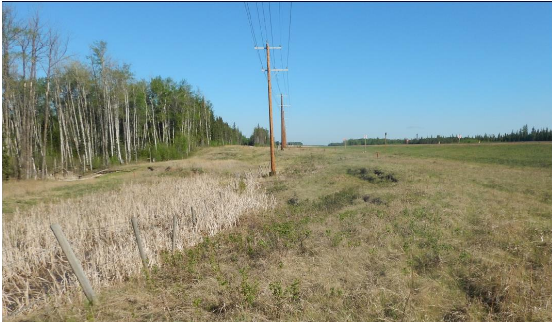
Photo No.4 –Looking north at the southern flank of upper and lower landslide blocks; note standing water within the flank and lateral shifting of existing fence; landslide is well vegetated.
