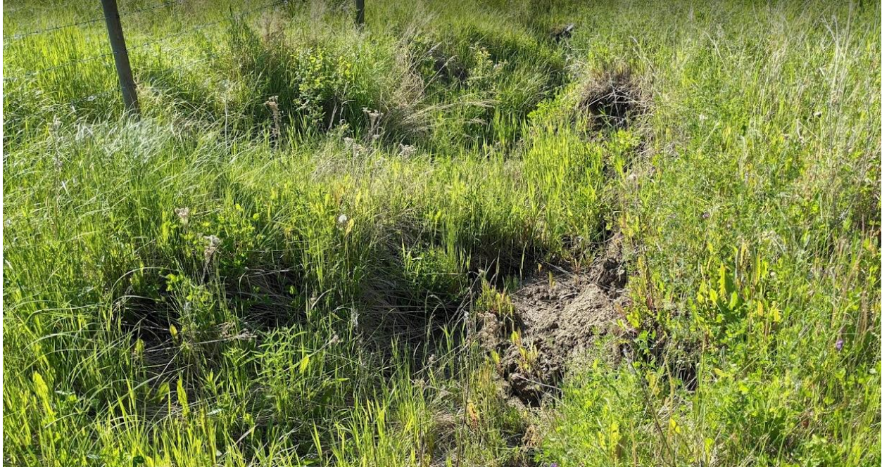
Photo No.3 – Erosion gully along Fischer Trail ditch (Looking South)
