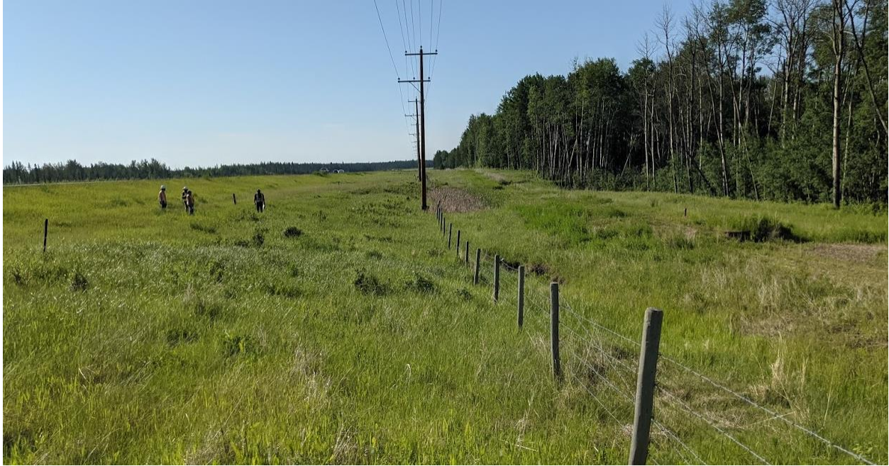
Photo No.1 – Head scarp crack of upper landslide block (Looking South)
