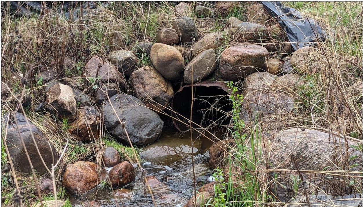
Photo No. 4 – Steady Water Flow at Culvert C1 outlet location
