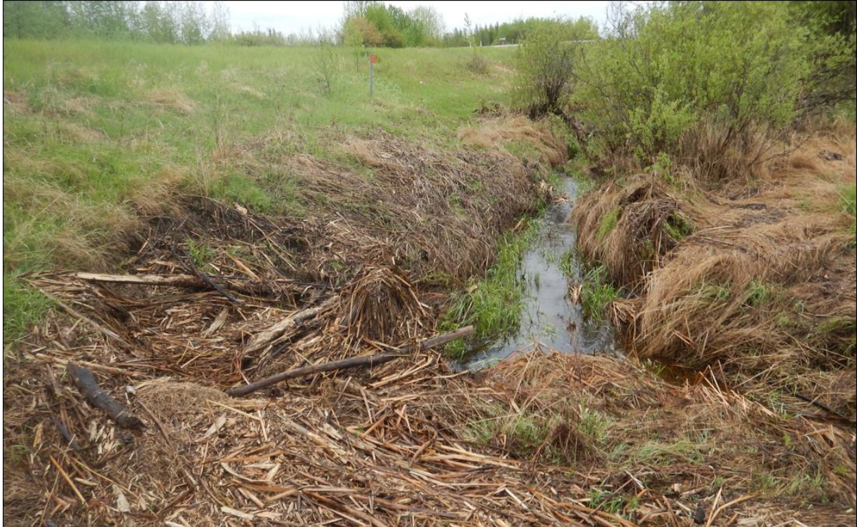
Photo No. 3 – Looking east towards CSP culvert C1 inlet
