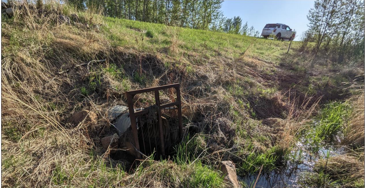
Photo No. 4 – Looking northeast at Culvert C1 inlet location
