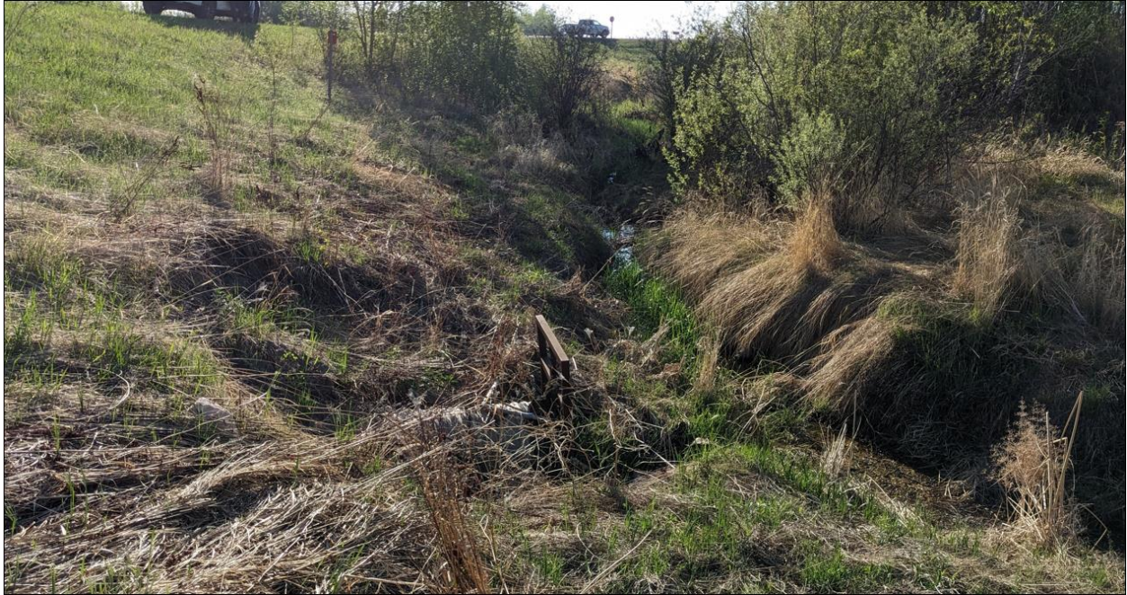
Photo No. 3 – Looking east towards CSP culvert C1 outlet
