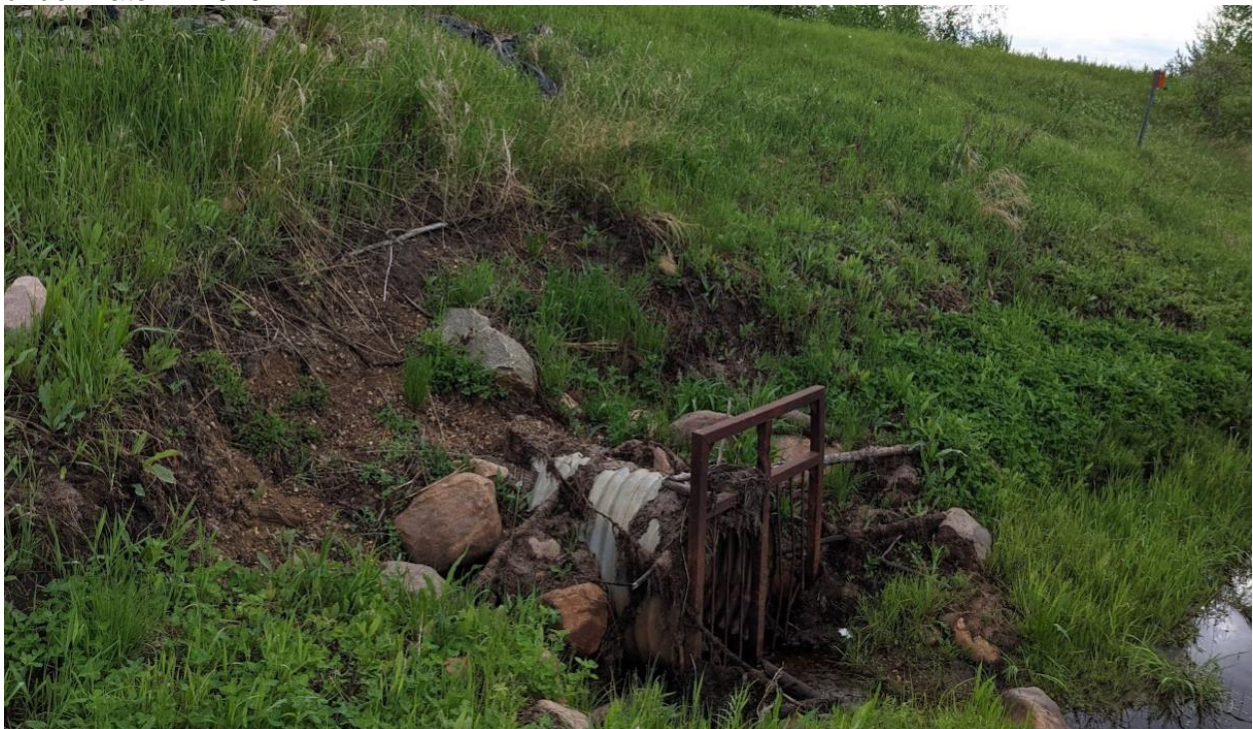
Photo No. 4 – Looking northeast at Culvert C1 inlet location
