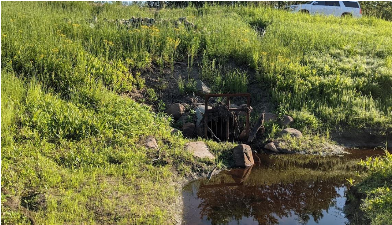
Photo No. 4 – Looking north at Culvert C1 inlet location
