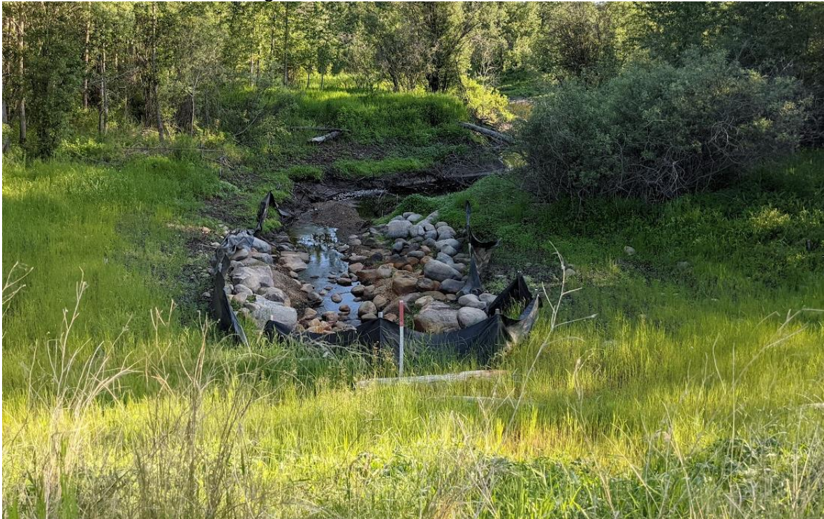
Photo No. 2 – Looking northeast at Culvert C1 outlet. Note that beaver dam, located downstream of the culvert outlet, was cleared so water was flowing freely along the channel
