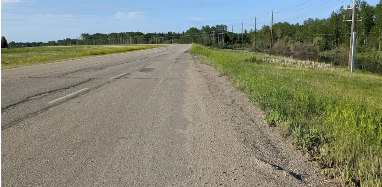
Photo No. 5 – Looking south at highway open cracks within the limits of the repaired area in 1997 (previously known as NC08-1)
