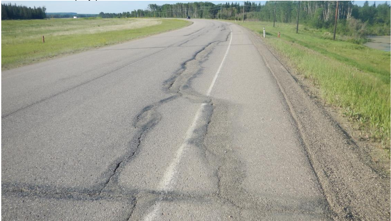
Photo No. 10 – Looking south at the northern flank of the new landslide (previously known as NC08-2); note exiting drop within the highway lane
