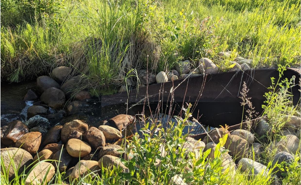
Photo No. 7 – Looking north at 900 mm diameter SWSP Culvert C2 outlet; heavy flow in 2021
