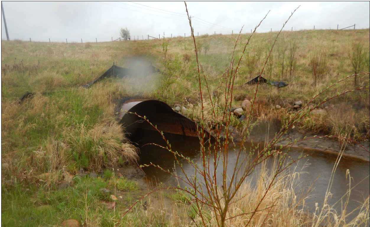
Photo No. 6 – Looking at the outlet of the SWSP centerline culvert
