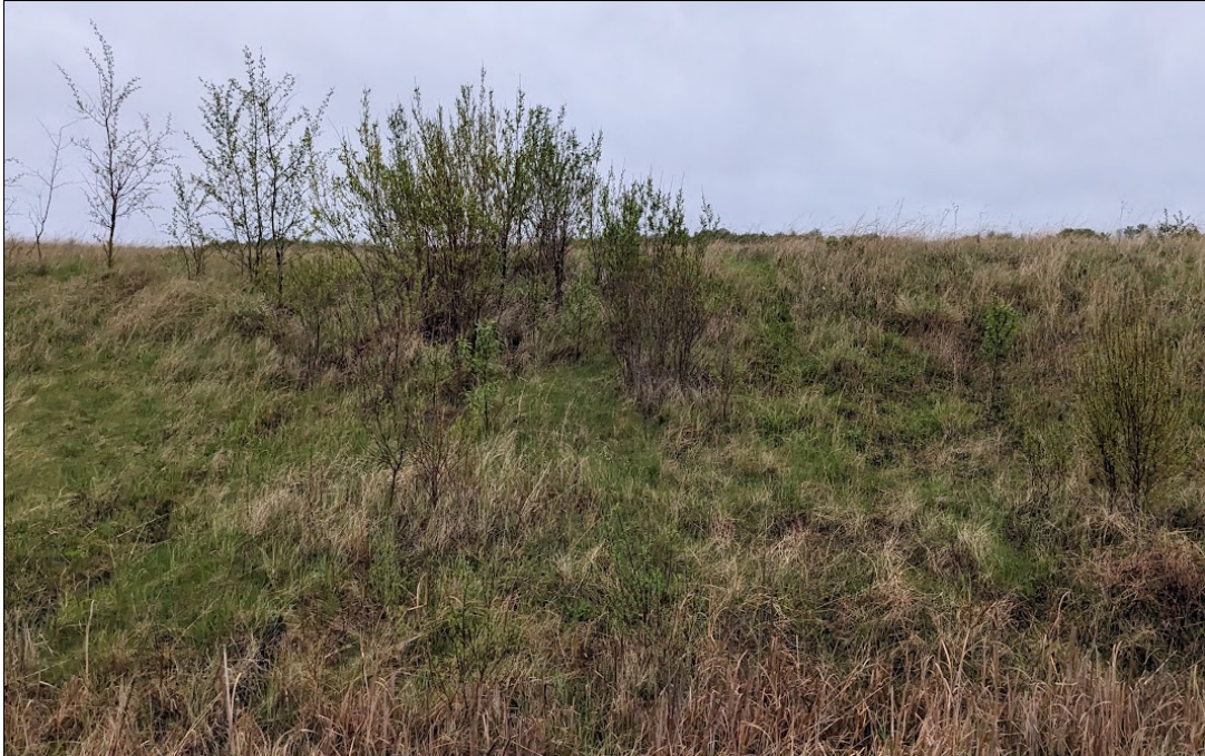
Photo No. 9 – Looking northeast at the backslope slump area observed in 2017; vegetation has grown within the slump area. Slump is not longer visible.
