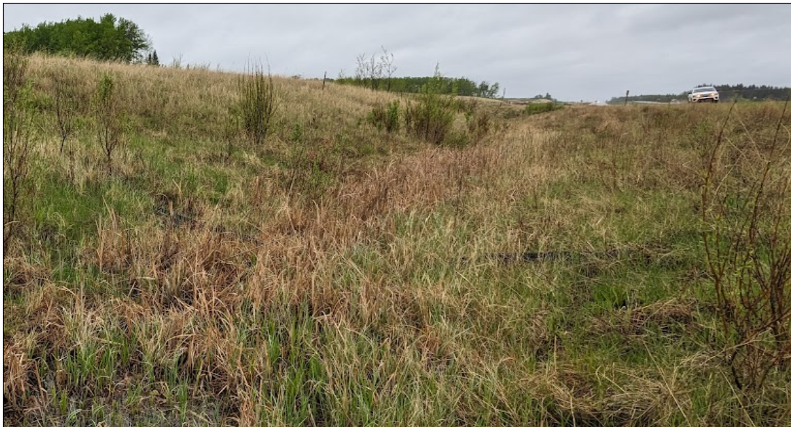
Photo No. 10 – South facing channel: Vegetation has grown within the upslope section of the channel and erosion is no longer visible
