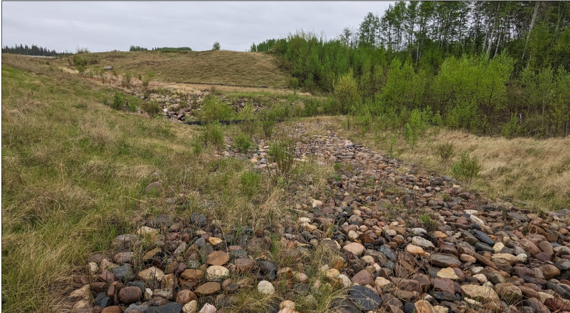
Photo No. 14 – Looking northeast along the riprap lined north facing drainage channel
