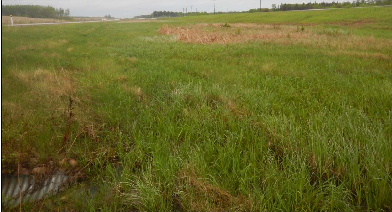
Photo No. 7 – Looking south at highway median. Heavy flow into the 600 mm diameter CSP culvert
