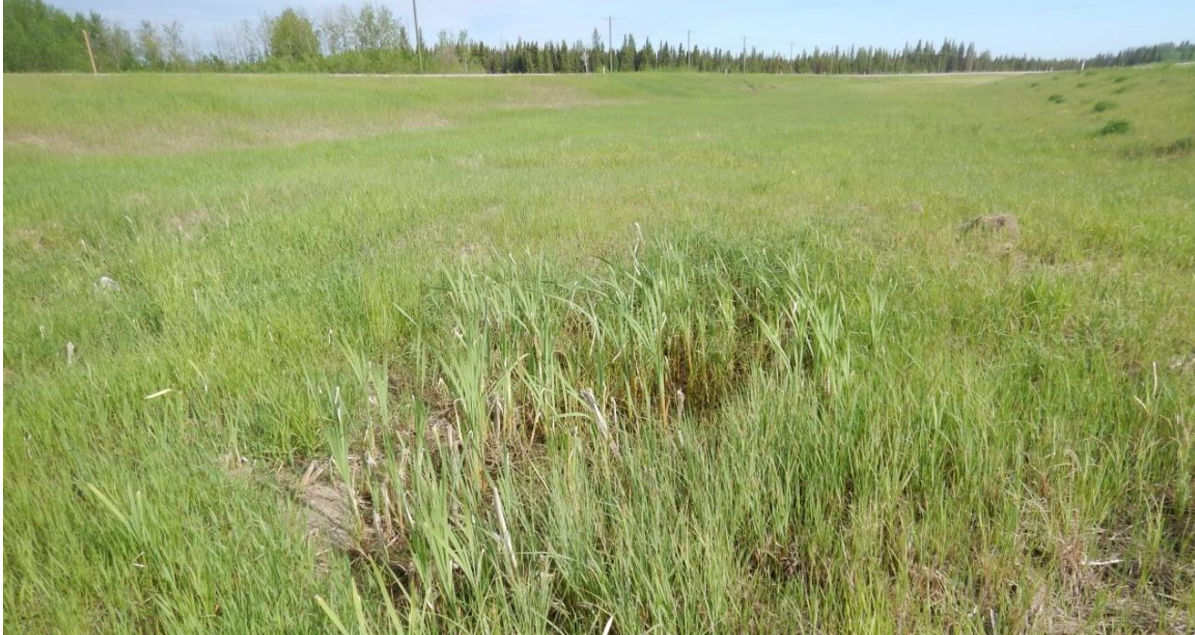
Photo No. 7 – Looking north at one of the sinkholes developed in the highway median
