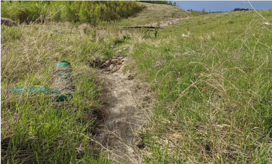
Photo No. 11 – Looking south at a gully approximately 900 mm wide x 400 mm deep; note vegetation is starting to cover the gully in this zone
