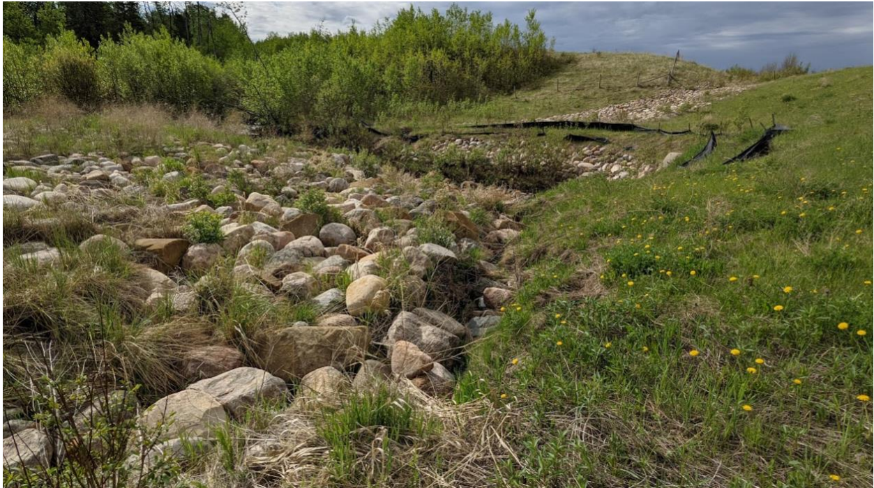
Photo No. 13 – Erosion gully developed on the west edge of the channel has been filled with riprap
