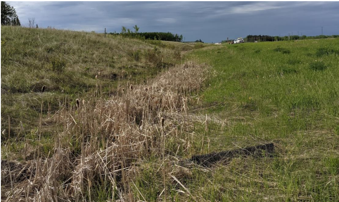
Photo No. 10 – South facing channel; looking at synthetic ditch barrier; note vegetation has grown and erosion in this area is no longer visible
