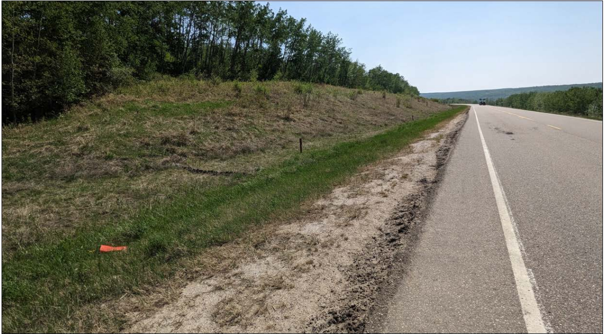
Photo No. 9 – Looking south at ditch and a gully lined with TRM
