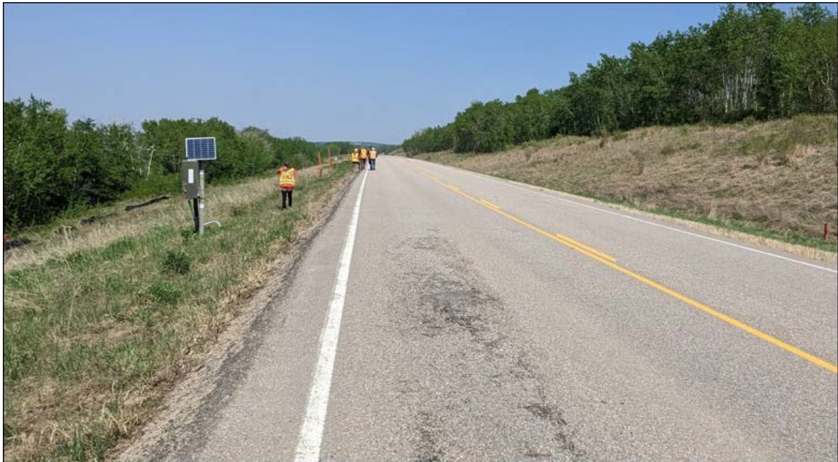
Photo No.6 - Looking at data logger DT1 installed at pile 146 location; vegetation grew at previously noted subsidence at the base of the data logger
