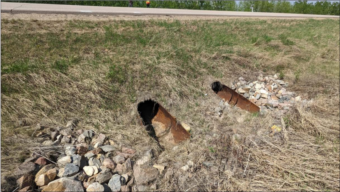
Photo No.3 - Looking at the twin culverts inlets; no flow
