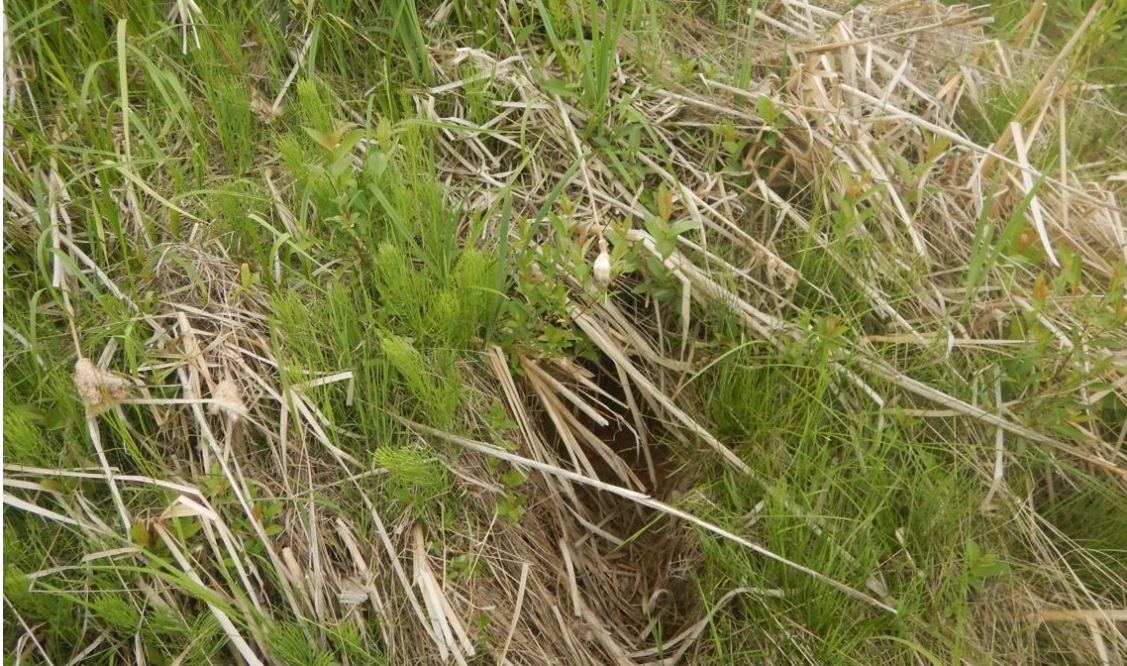
Photo No.5 - Looking at culvert C2 inlet; no flow in 2021
