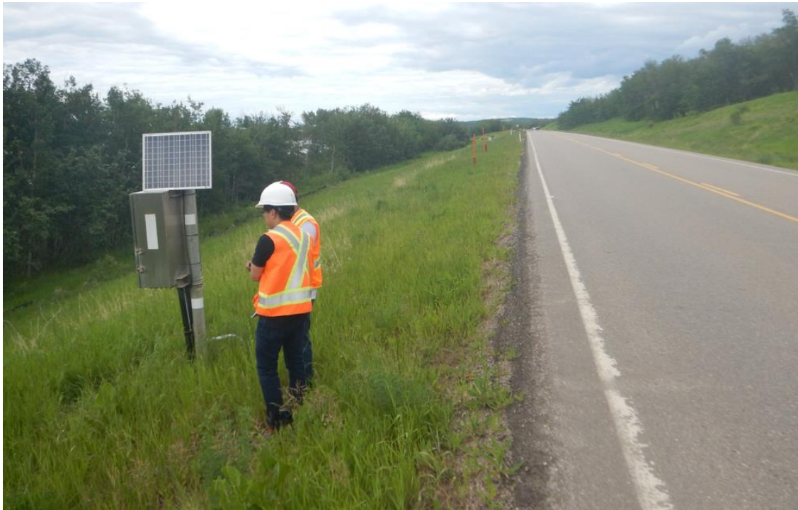
Photo No.6 - Looking at data logger DT1 installed at pile 146 location; vegetation grew at previously noted subsidence at the base of the data logger
