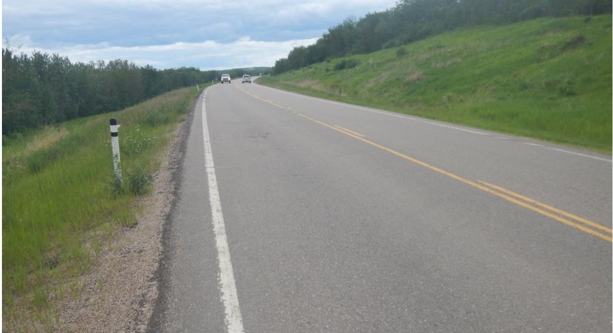
Photo No. 1 - Looking north at highway surface; no reflective cracks or dips noted in 2021
