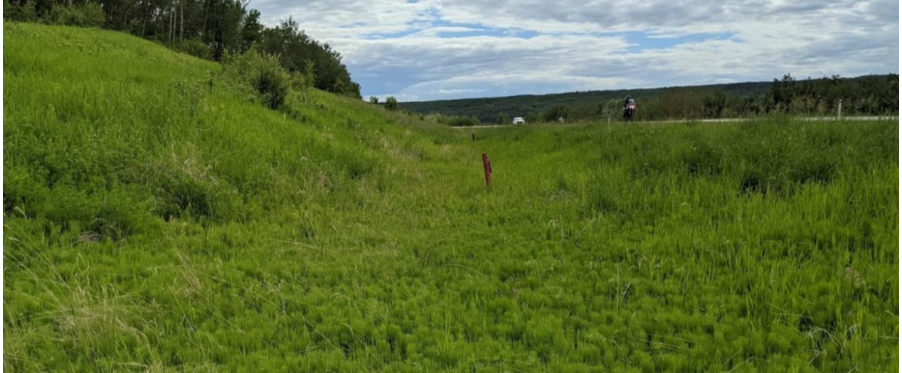
Photo No. 9 – Looking south at TRM lined ditch; note lush vegetation but no flow in 2021
