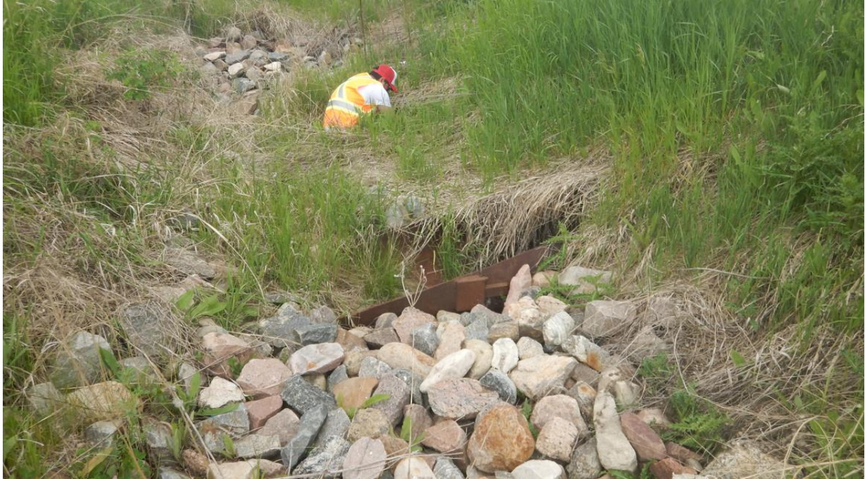
Photo No.3 - Looking at the twin culverts inlets; no flow in 2021
