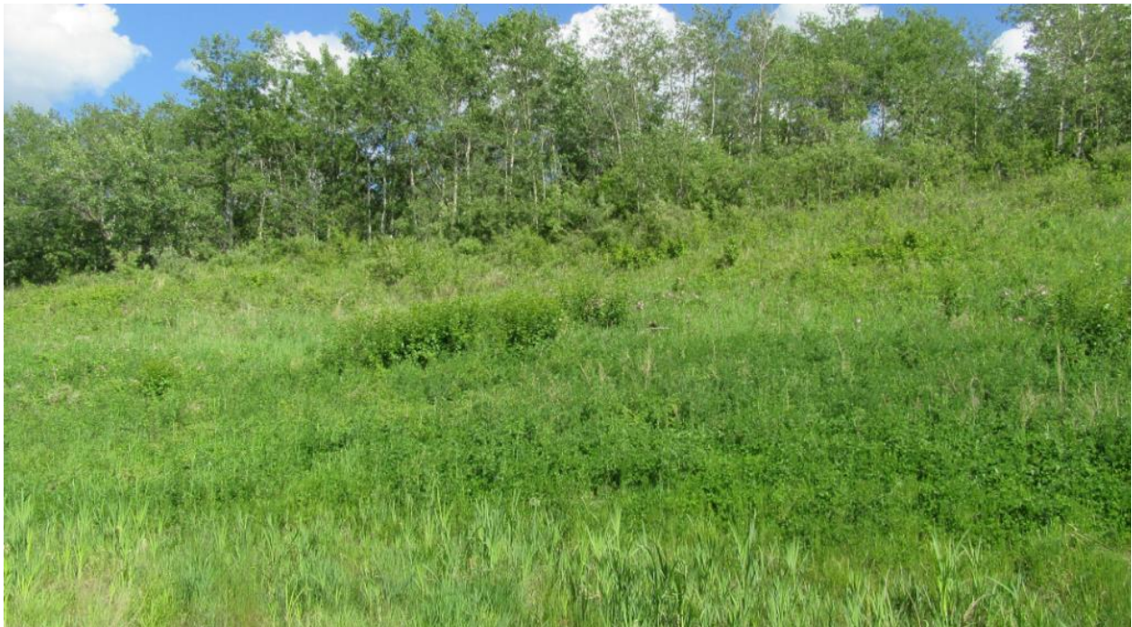
Photo No.4 - Looking east at backslope seepage zone; vegetation grew between 2018 and 2019
