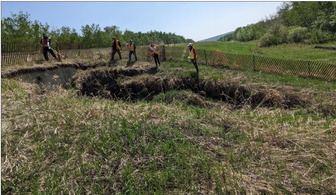
Photo No. 4 – Looking south at the slump downslope of the pile wall location
