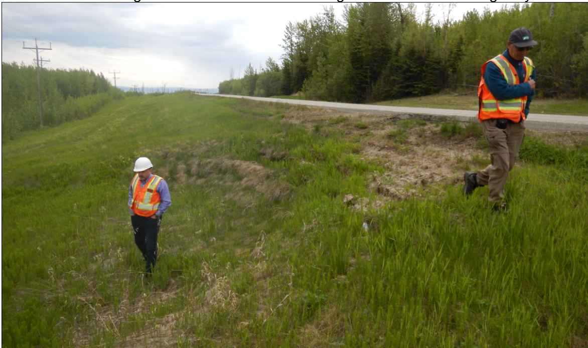
Photo No. 4 – Looking east at the landslide developed on the highway side slope; head scarp crack measured at 4.4 m from the white line (same as measured in 2022)
