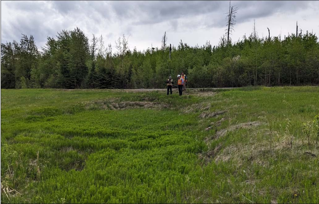
Photo No. 5 – Looking southeast at the head scarp crack of landslide mass; a distinct toe roll noted at the bottom of the slope; more vegetation grew within the landslide mass
