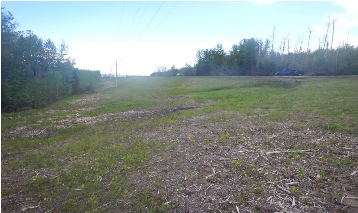
Photo No.5 – Looking east at the landslide mass and a distinct toe roll at the bottom of the slope
