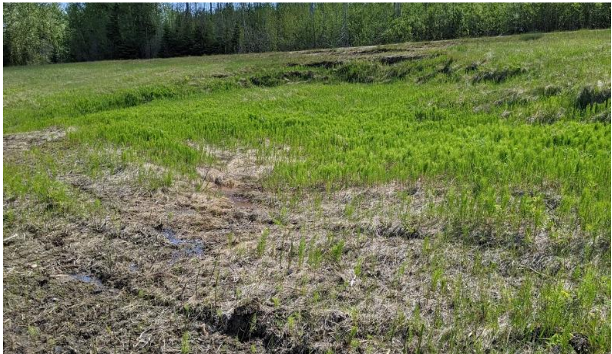
Photo No.6 – Looking southeast at the landslide head scarp crack and east flank
