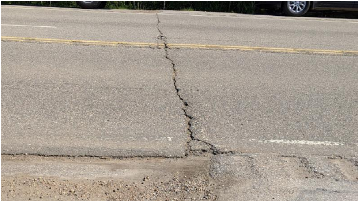
Photo # 4 Looking north at Crack D (East end of treated section)
