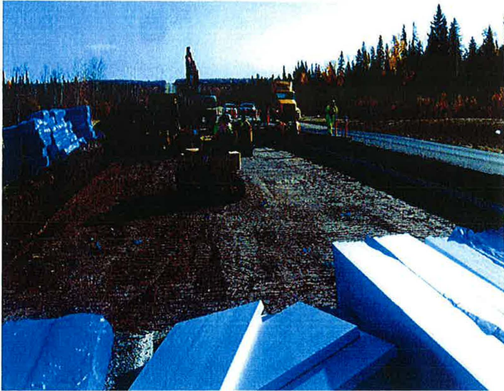
Picture -15 Subgrade Excavation for Frost Heave Repair (km 39.459 to km 39.545)
