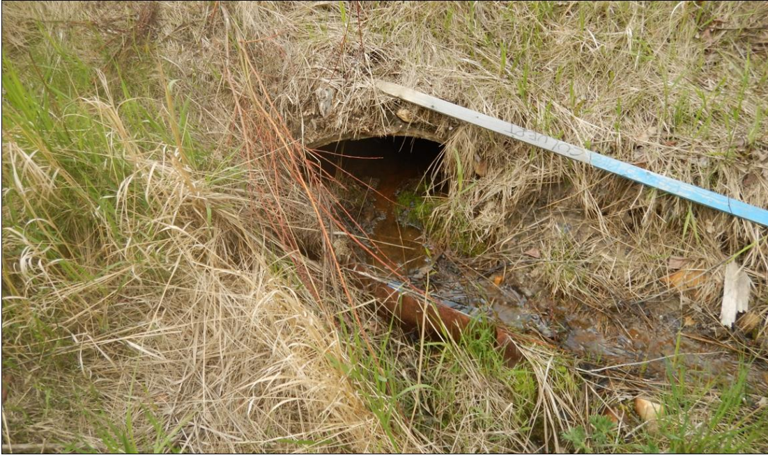
Photo No. 9 – Looking at 800 mm CSP culvert outlet
