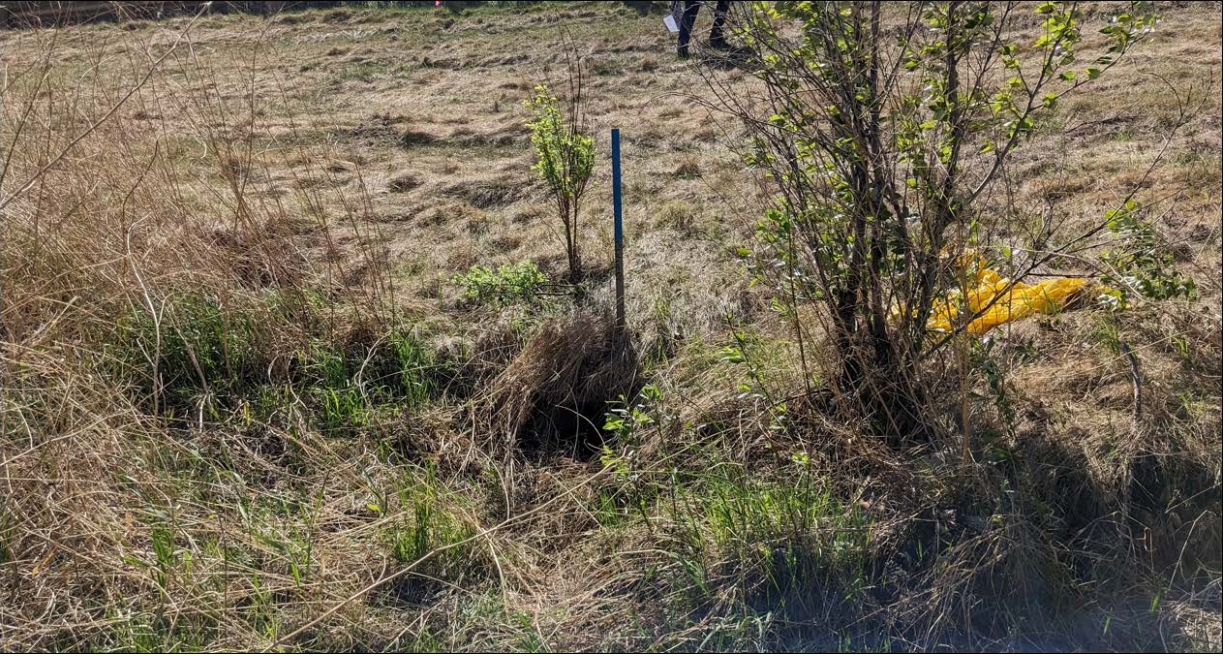
Photo No. 9 – Looking at 800 mm CSP culvert outlet.
