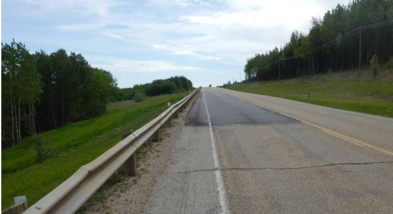
Photo No. 1 – Looking east toward the landslide and 2021 ACP patch; more vegetation grew on the highway side slope
