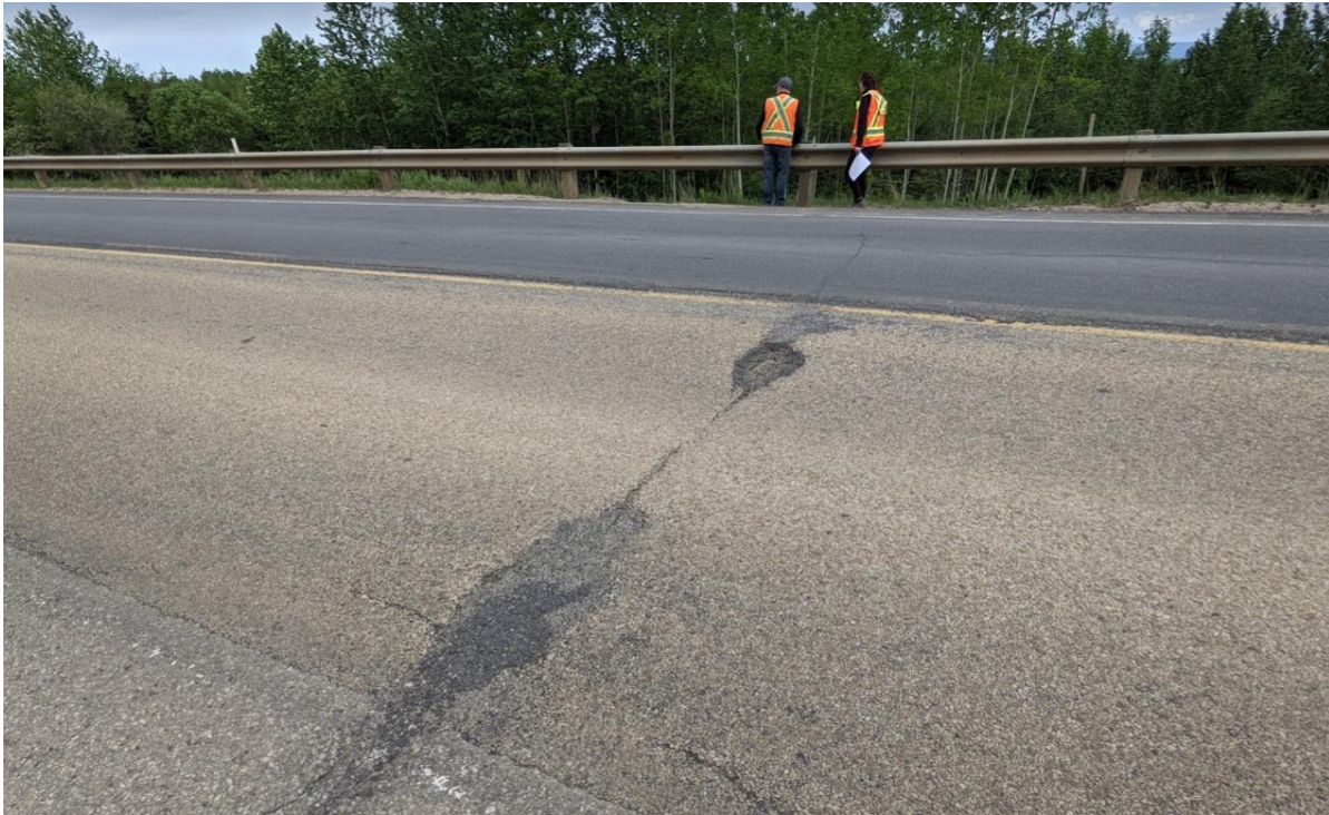
Photo No. 9 – Looking north at patched potholes on the east bound lane
