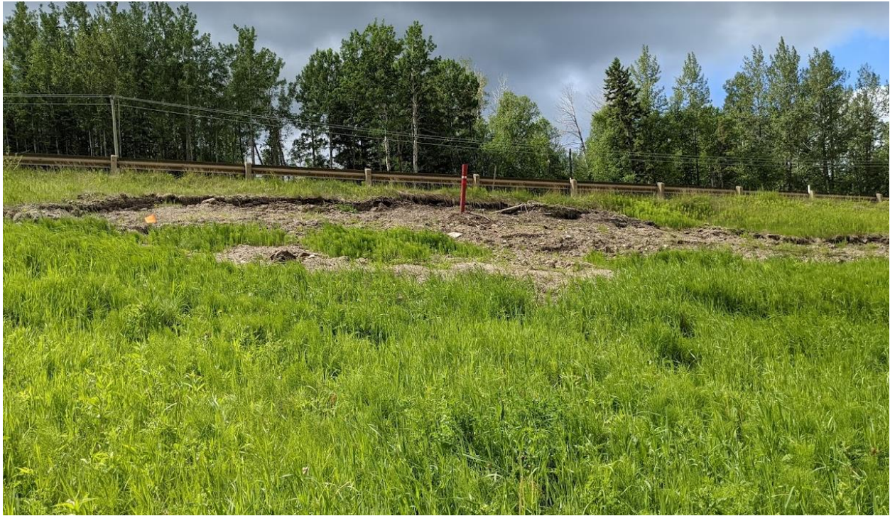
Photo No. 9 – Looking south at active landslide area
