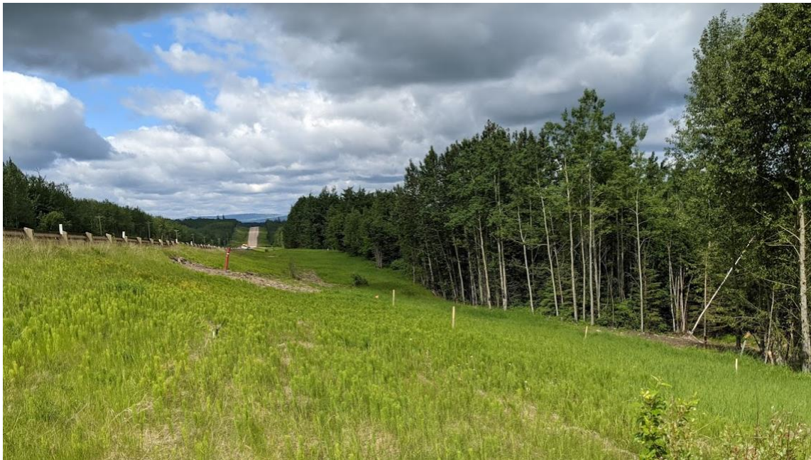
Photo No. 8 – Side slopes near the landslide head scarp
