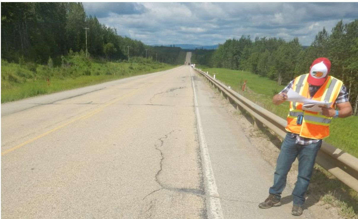
Photo No. 6 – Looking west at the middle section of the landslide block;
