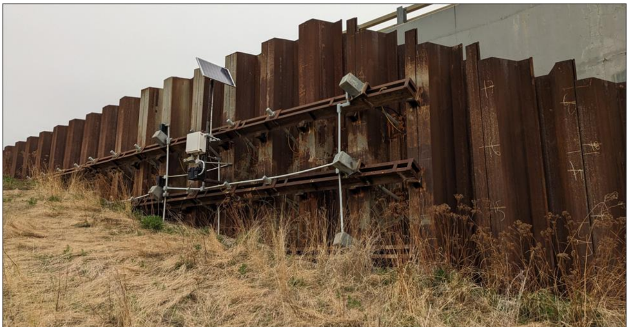
Photo 10. Datalogger enclosure and solar panel installed on Sheet Pile Wall B
