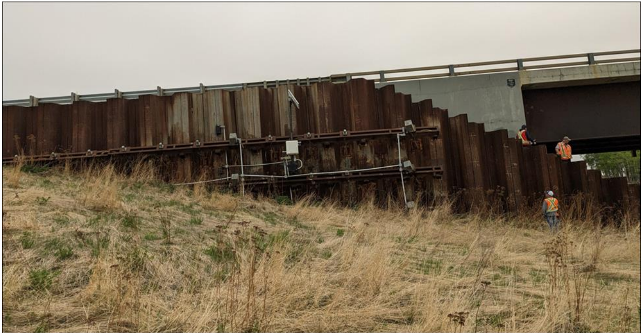
Photo 9. Well grown vegetation along the 6H:1V north facing slope
