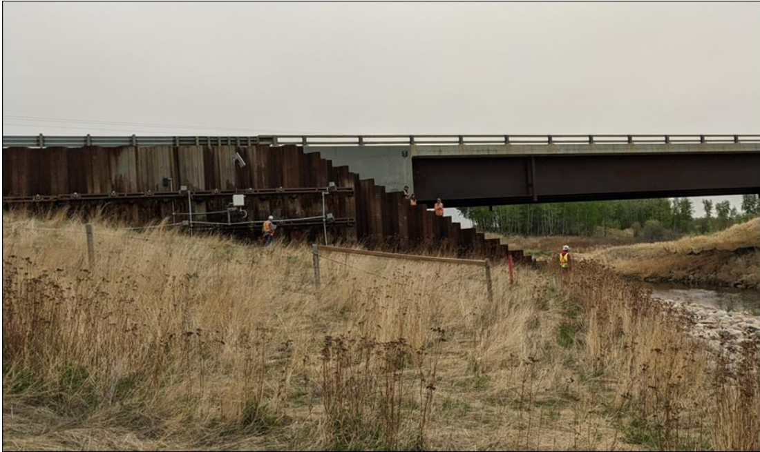
Photo 11. Well grown vegetation on both sides of the barbed Wire Fencing Installed on 6H:1V north facing slope
