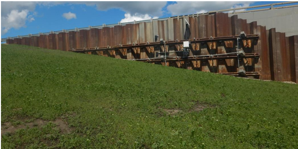
Photo No. 7 – Vegetation growing nicely along the newly graded 5H:1V north facing slope
