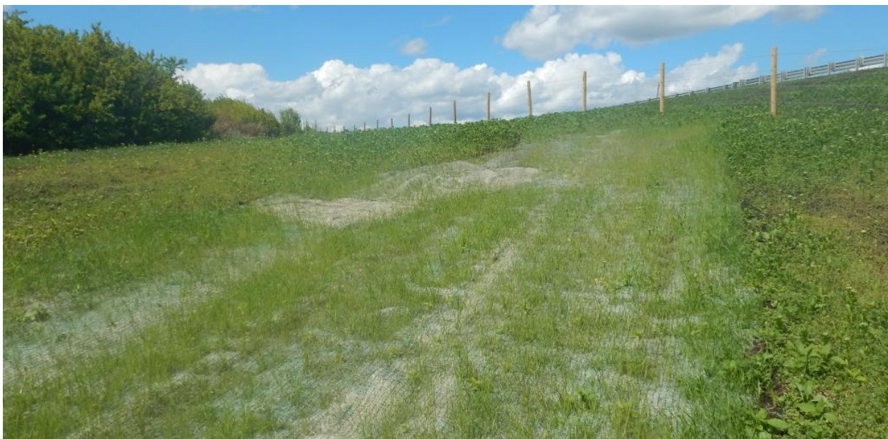
Photo No. 9 – New Type C TRM and Barbed Wire Fencing
