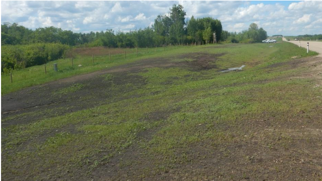
Photo No. 2 – Looking north at some rill erosion developing south of the highway ditch
