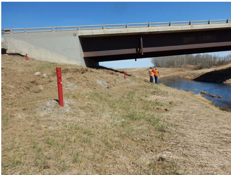
Photo No. 10. - Looking east at the tension cracks of a slump developed within the landslide mass near the bottom of the slope
