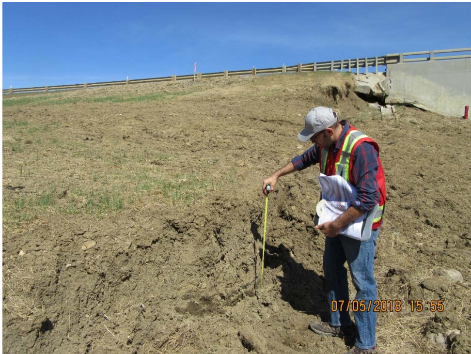
Photo No. 2. - Signs of seepage from the landslide head scarp crack (Looking East)
