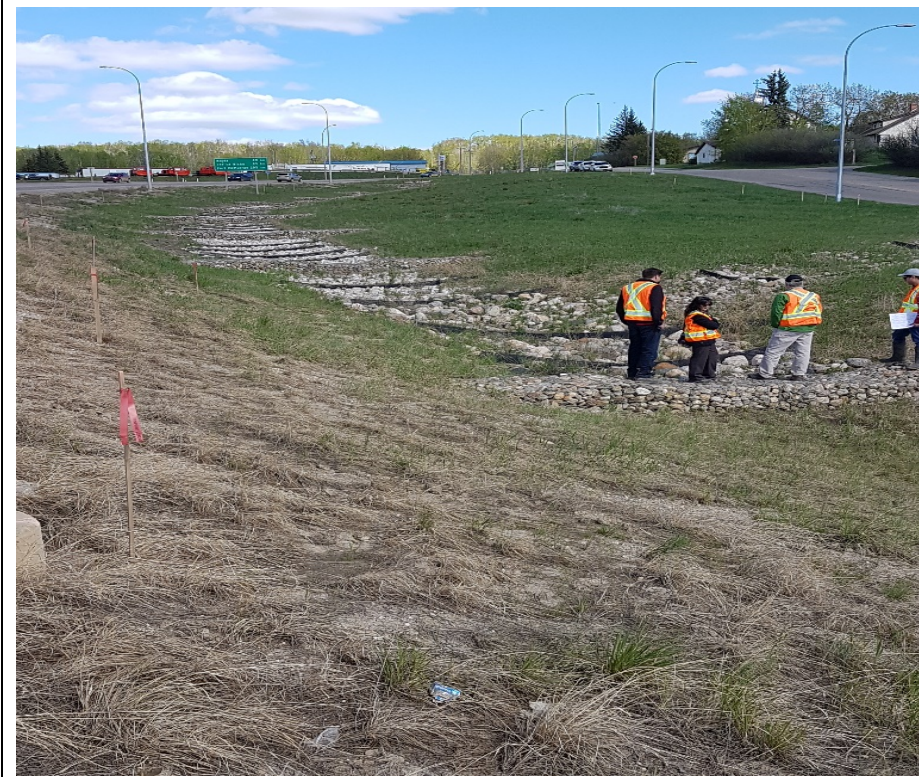
Photo #3. Hwy 55 South Ditch: Looking east at the existing riprap channel
