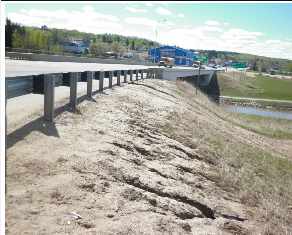
Photo #11. Looking west at the northeast corner of the intersection of Hwy 55 and 813. Bare vegetation and erosion rills in this area
