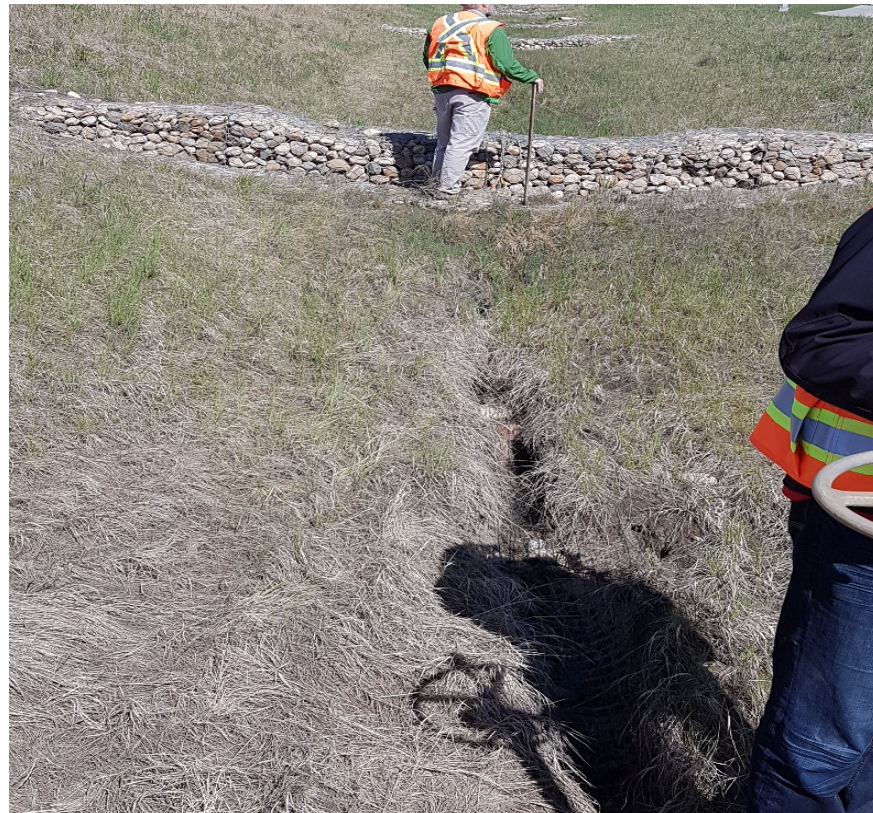
Photo #8. Hwy 55 south ditch: looking east at erosion gully between G 12 and the spill containment ditch block
