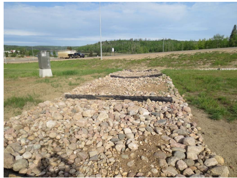
Photo 7. Looking northwest at the existing Class 1 M Riprap lined swale extending from the end of the concrete curb and gutter along the north edge of 50 Avenue to the south ditch of Hwy 55; note the presence of bare ground around the swale and areas bare or riprap within the swale.
