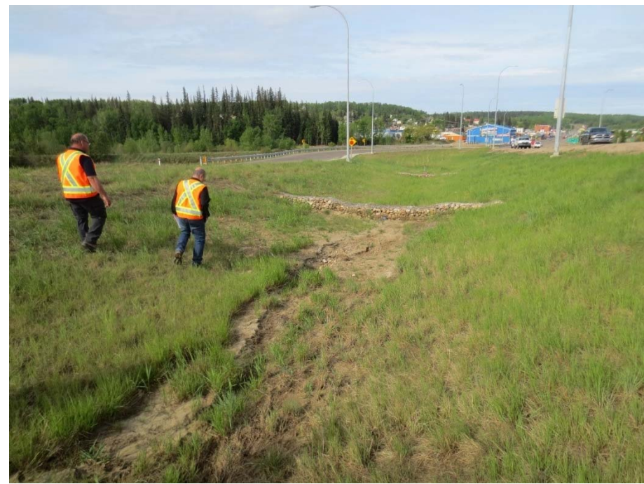
Photo 9. Hwy 55 south ditch: looking west at the ditch between G10 and G11; the ditch bottom is bare of vegetation and signs of erosion were noted in this area
