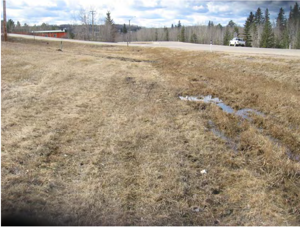
Photo 7 – Ponding water in the south highway ditch- Looking west
