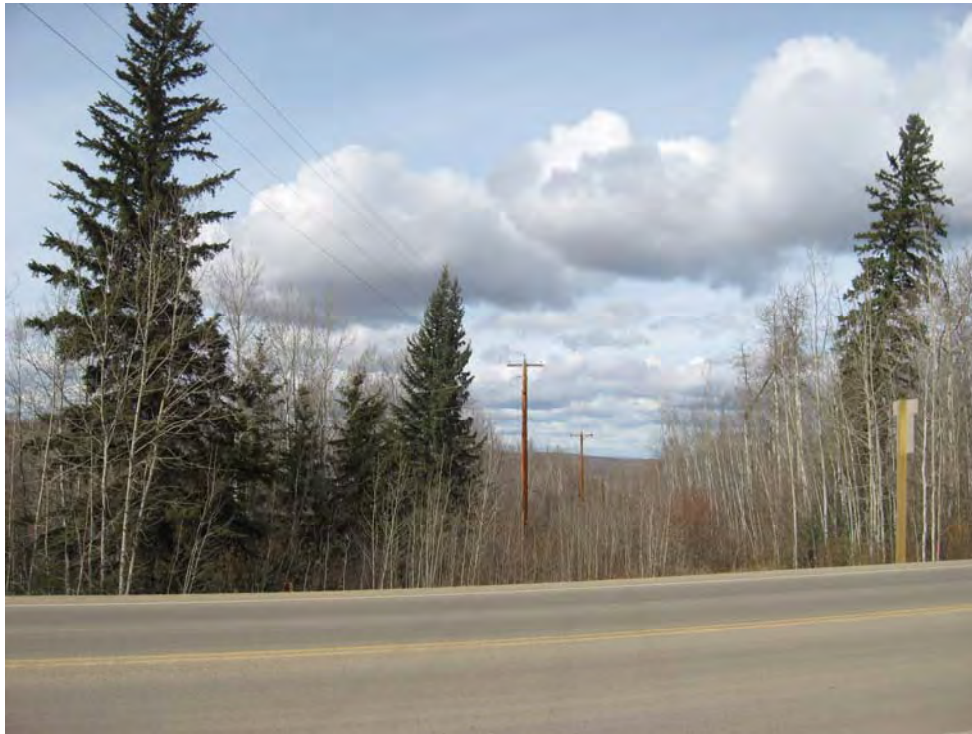
Photo 15 –Looking north at tilting trees downslope of the highway
