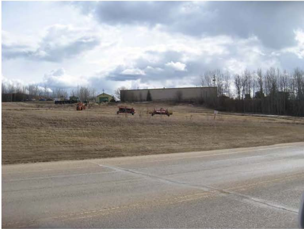
Photo 3 - Looking south towards the highway backslope
