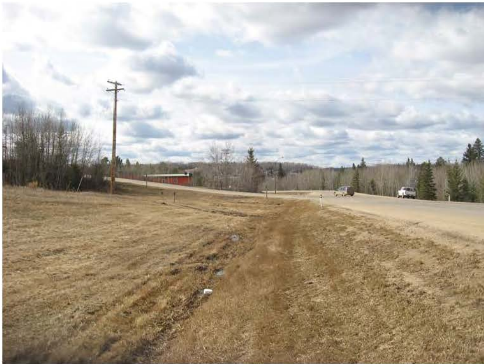
Photo 4 - Looking west at the highway south side slope and backslope
