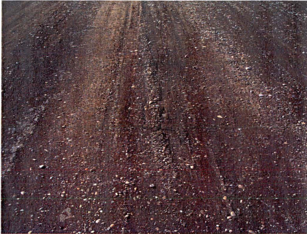
Photo 3 - Looking at the Roadway Surface at the Distress Area.
