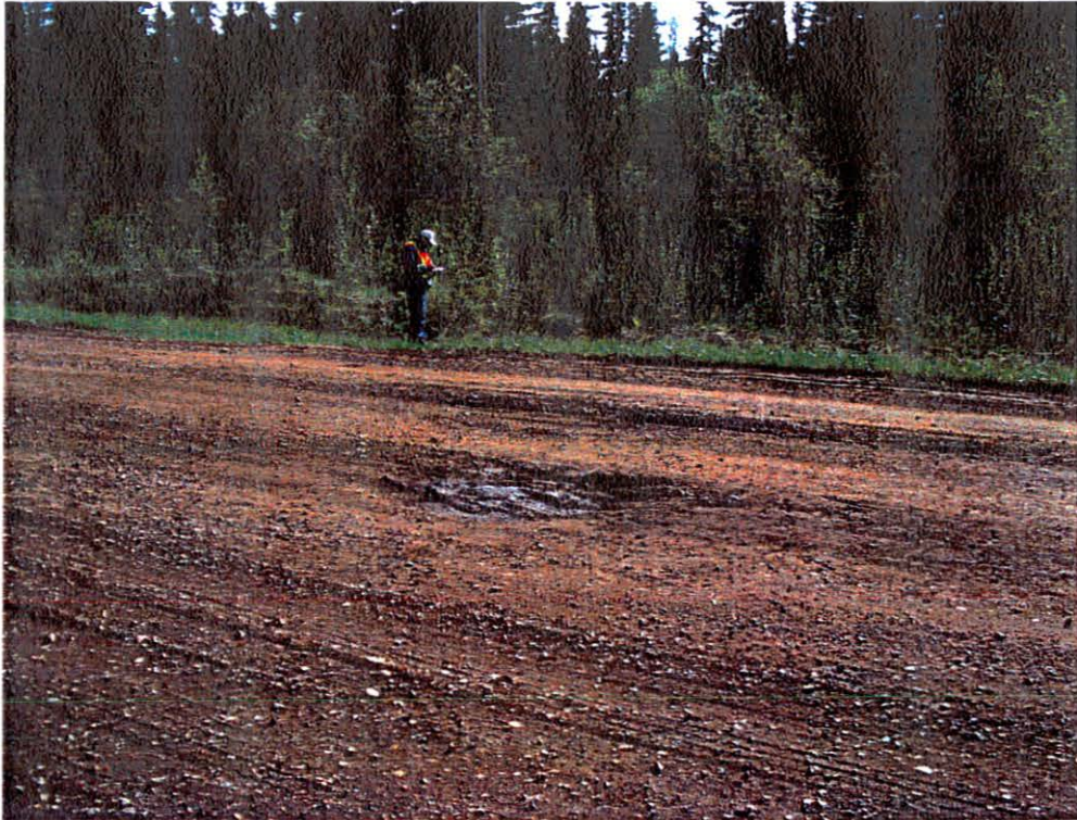
Photo 1 - Looking East at the Soft Spot.
