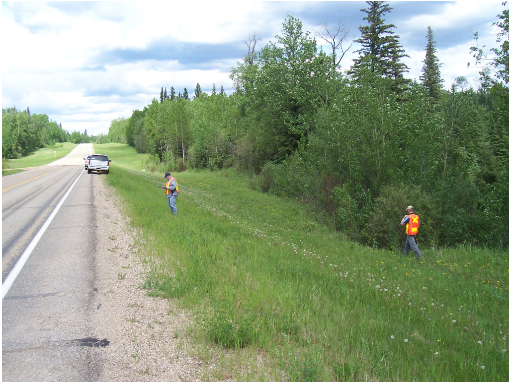
Photo #1 Looking North at the highway side slope
