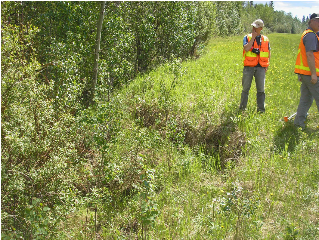
Photo #2 Looking south at the slide vegetated head scarp
