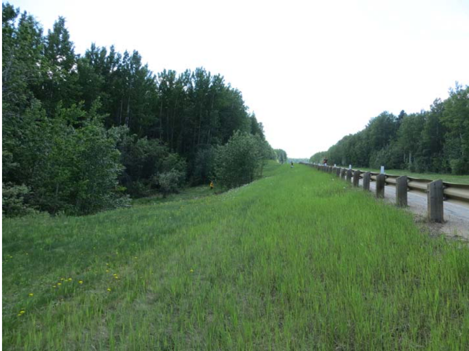
Photo#3 Looking south east at the landslide mass
