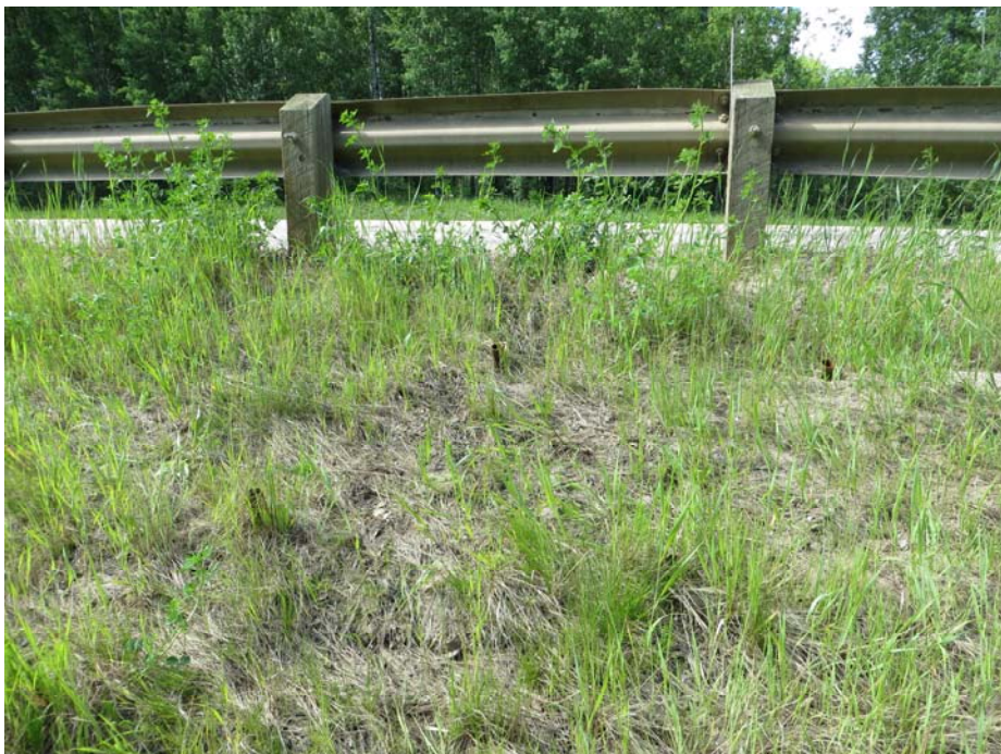
Photo#4 Looking northwest at the soil nails installed above the main headscarp
