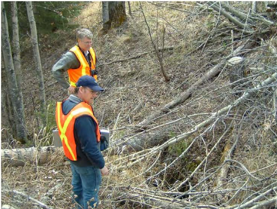
Photo 5 & 6 Looking at the Gully at km 10.45, May 2, 2006.
